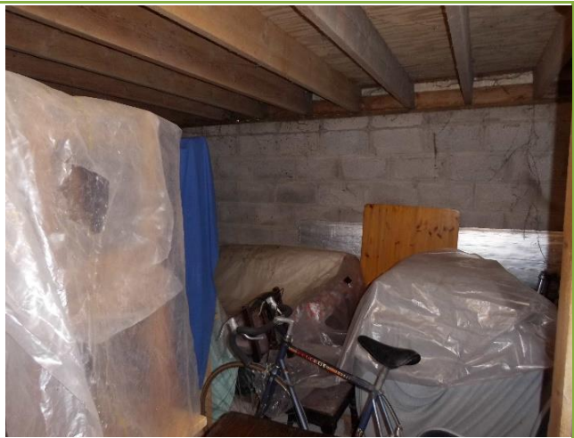
Interior (storage area)
