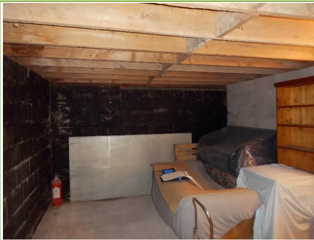
Interior (storage area)
