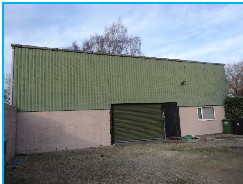
Fig 5 Image of outbuilding showing robust character, high eaves and ridge, with compacted hardcore apron and impermeable paths.
