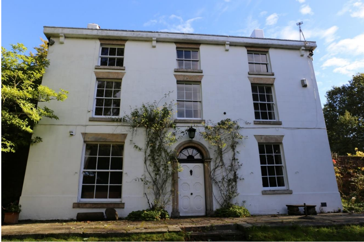
Plate 9: Front elevation of Fisher House
