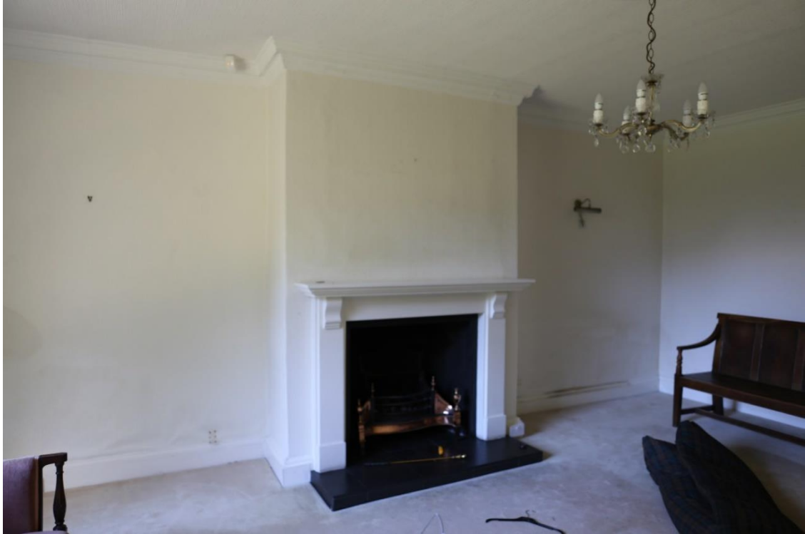
Plate 16: Chimney breast and fireplace in ground floor parlour
