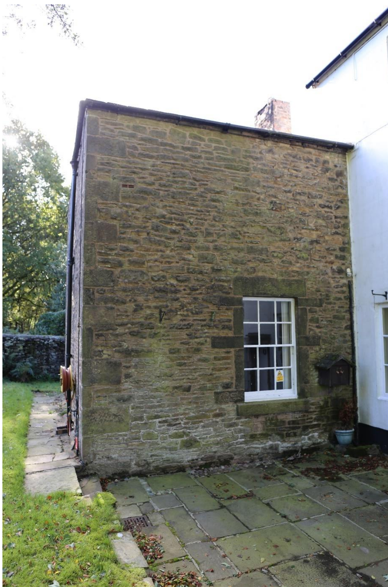
Plate 35: The eastern service wing, facing south-east
