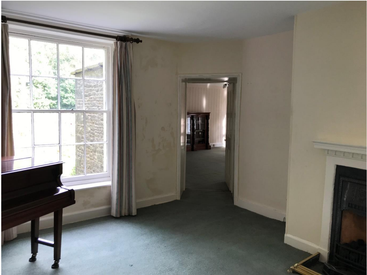
Plate 39: The library room on the first floor has been connected into the landing in the main dwelling
