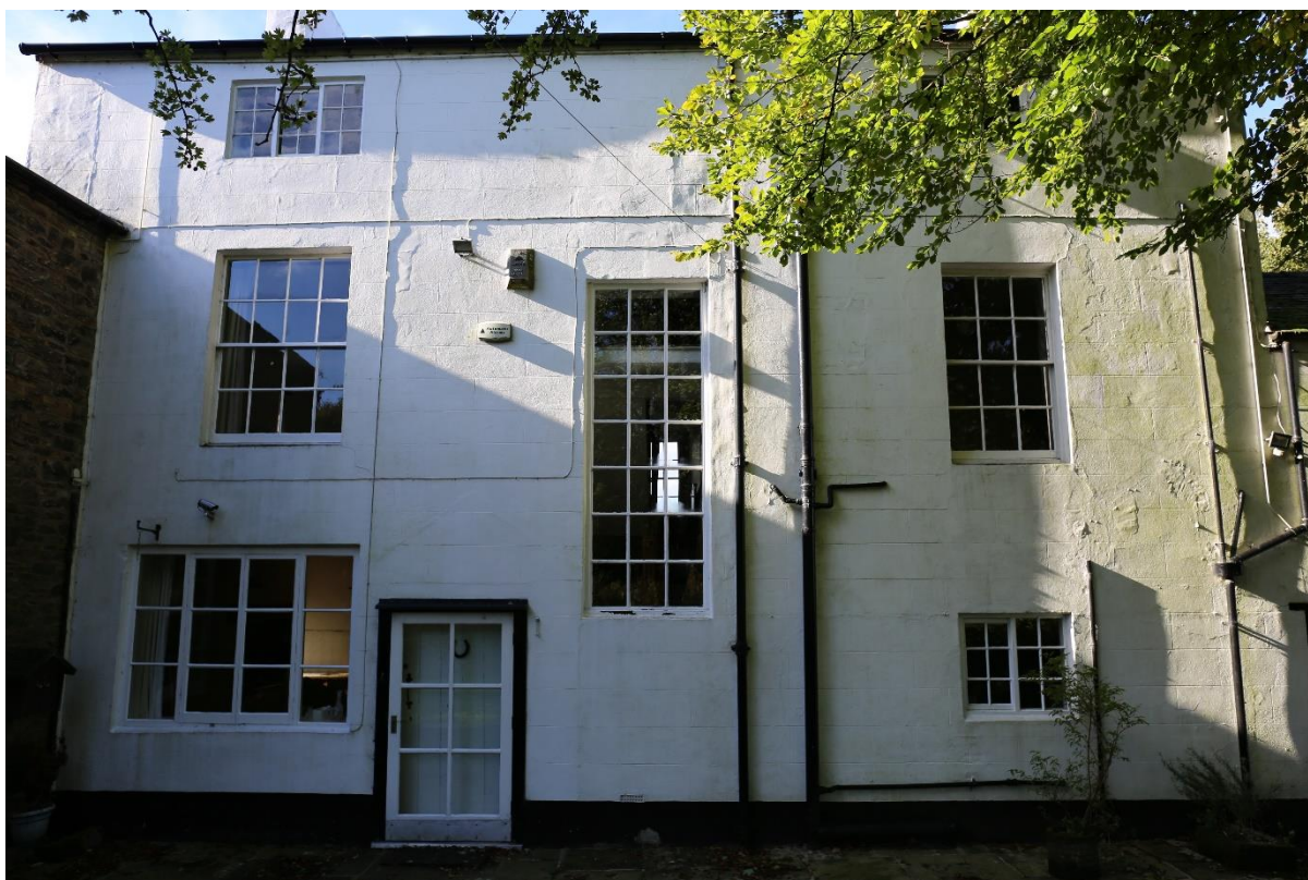
Plate 12: Rear elevation, Fisher House
