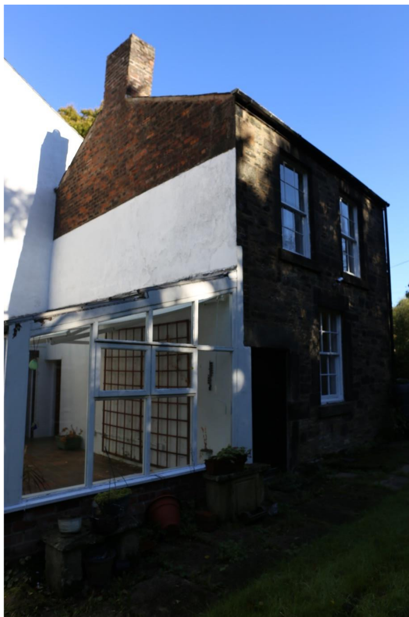
Plate 42: UPVC conservatory / sunroom as built against the servants' wing
