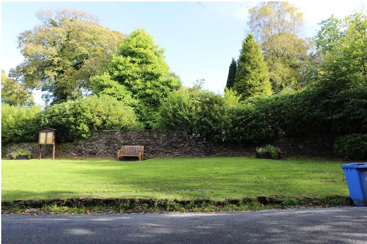
Plate 8: Stone curtain wall screening Fisher House from the village green and highway, facing north-east towards the property
