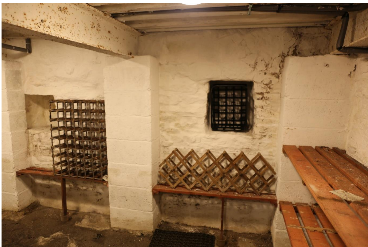
Plate 27: Cubby holes in the basement walls
