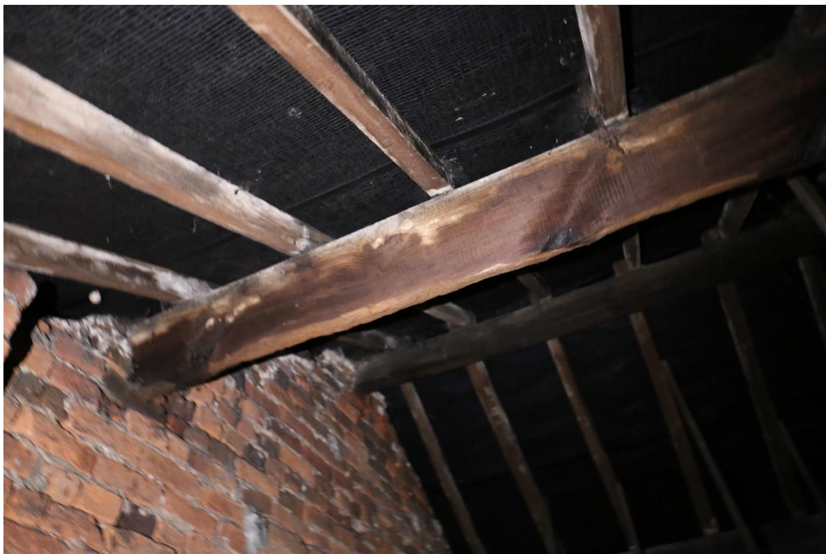
Plate 11: Modern roof frame over Fisher House
