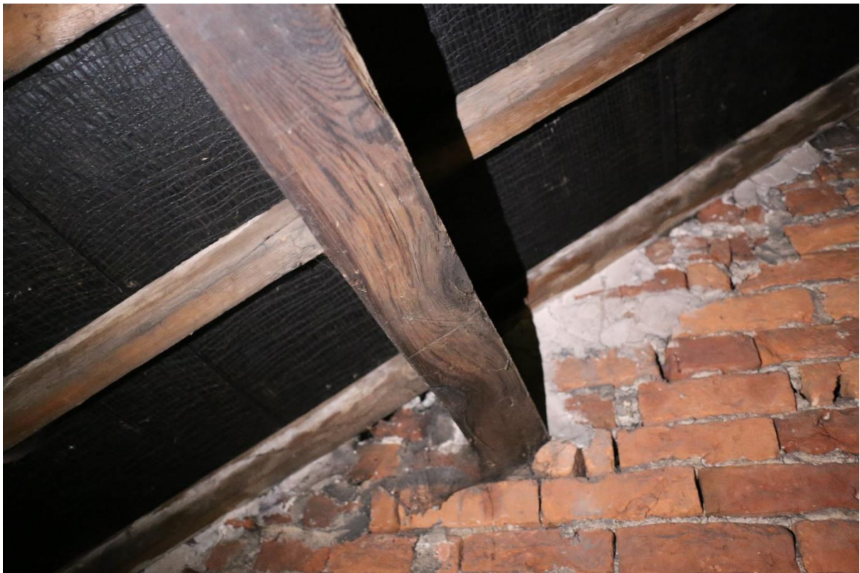
Plate 10: Modern roof frame over Fisher House
