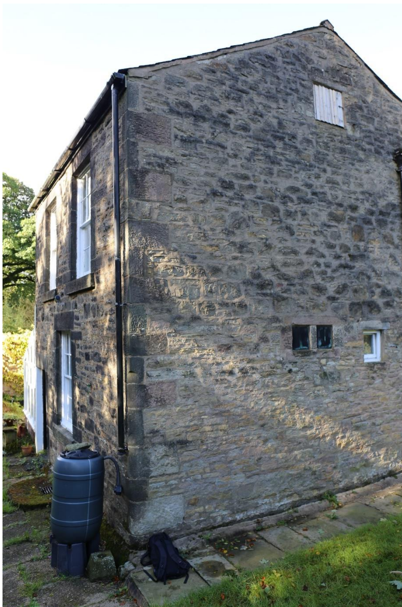
Plate 36: The eastern service wing, facing south-west
