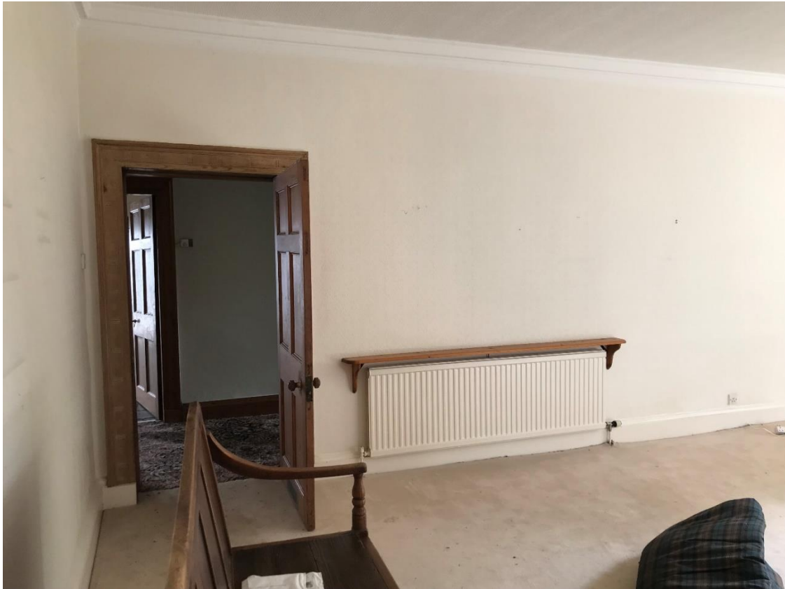
Plate 21: First floor bedroom showing disconnect between door frame and skirts, suggesting some redesign.
