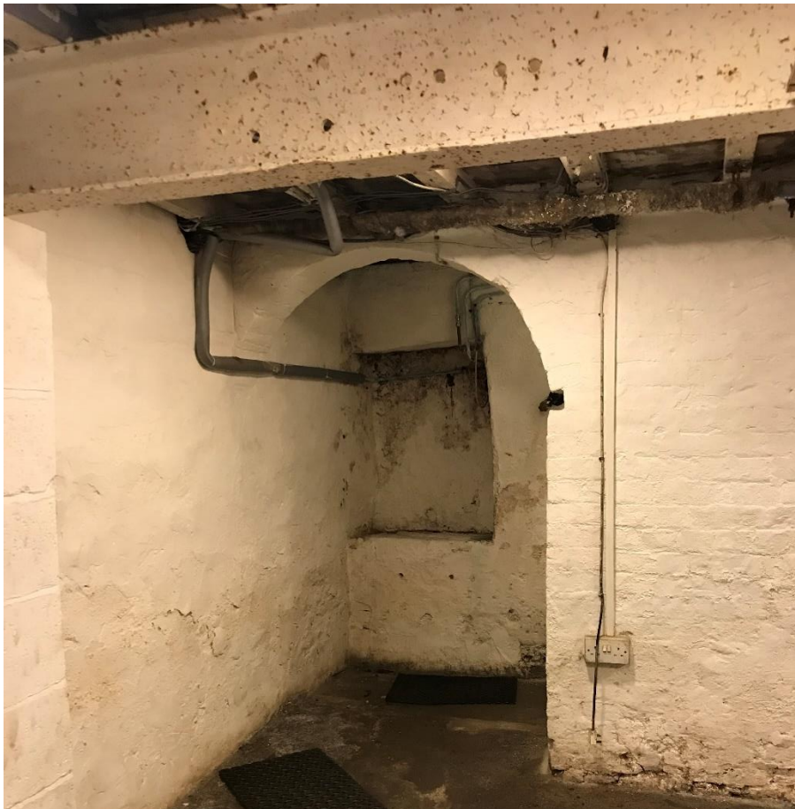
Plate 26: Original features in the basement include arched openings
