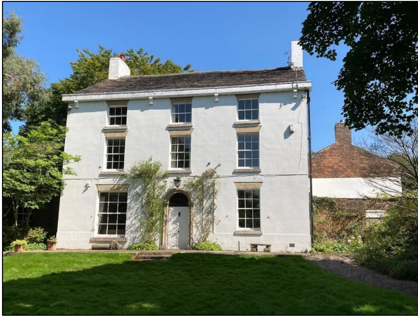
Photograph 1 showing the exterior of the building
