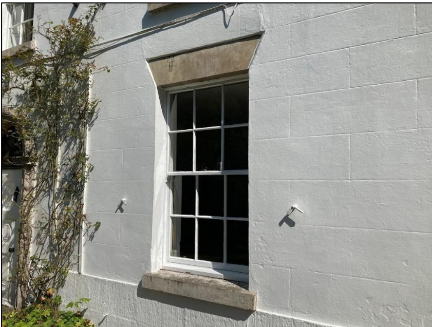
Photograph 5 showing one of the timber window frames
