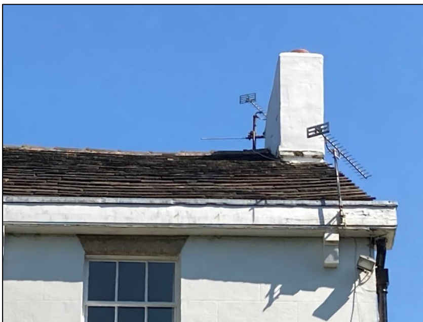
Photograph 7 showing the stone flag section of the roof
