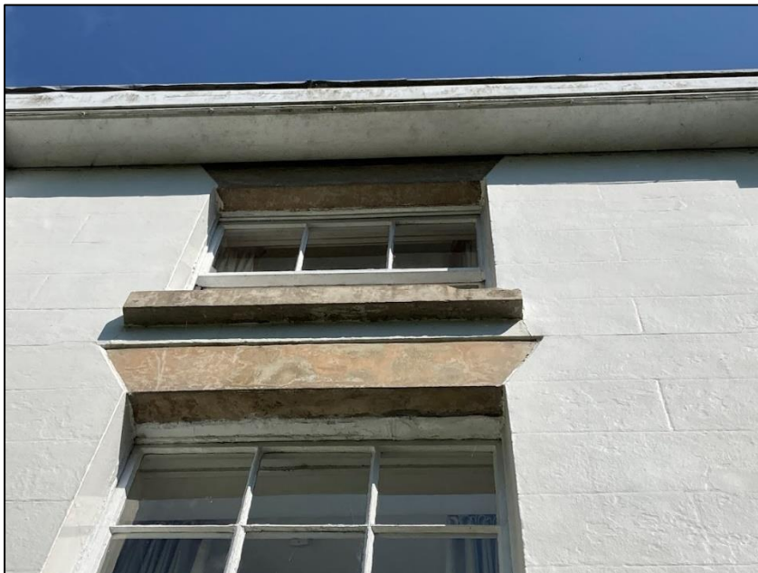
Photograph 13 showing the box guttering
