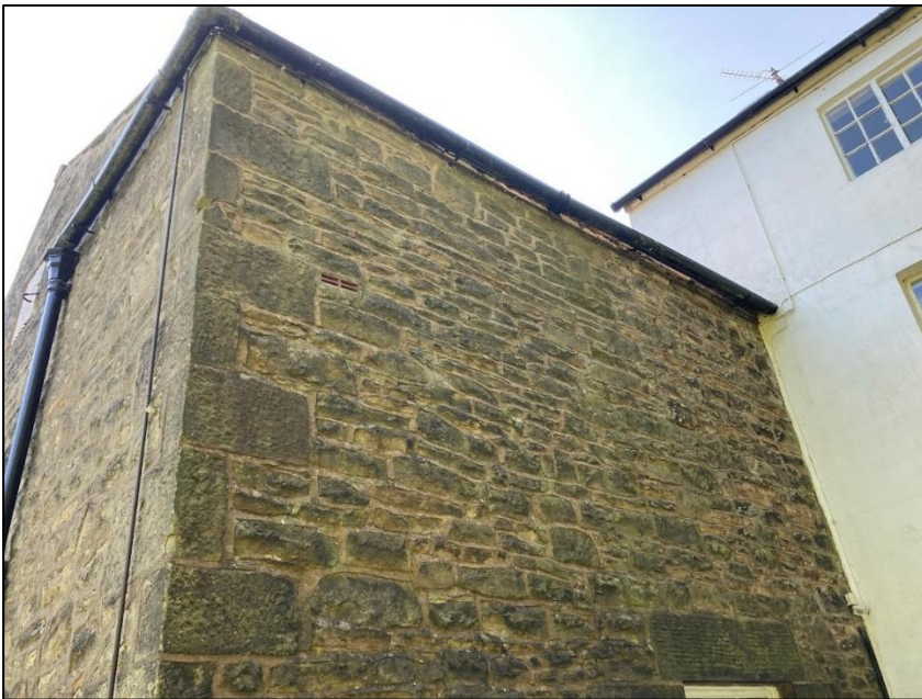
Photograph 3 showing the exterior of the building
