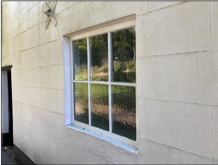
Photograph 6 showing one of the timber window frames
