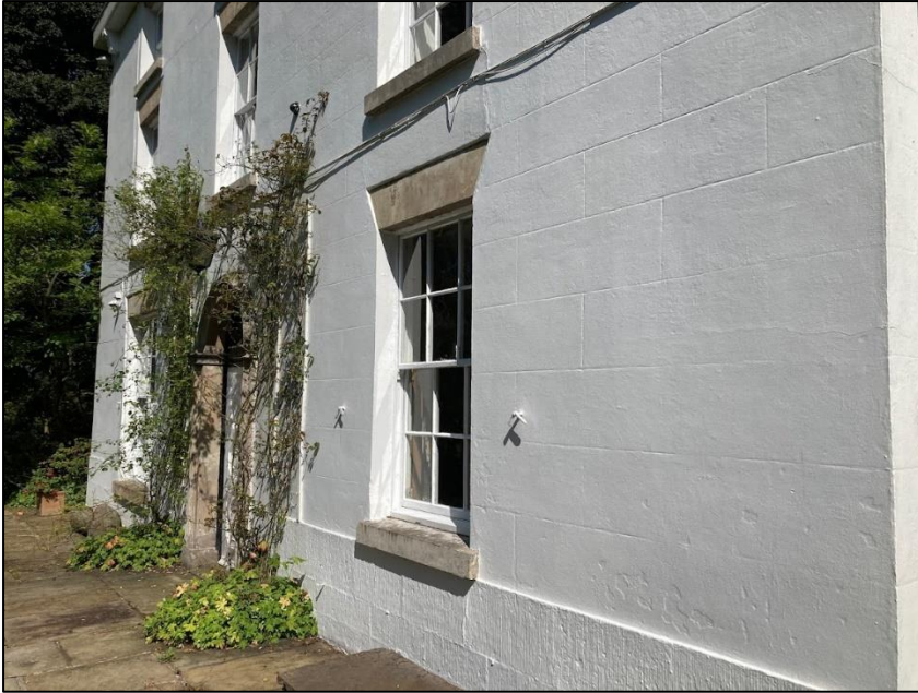
Photograph 2 showing a section of the rendered exterior
