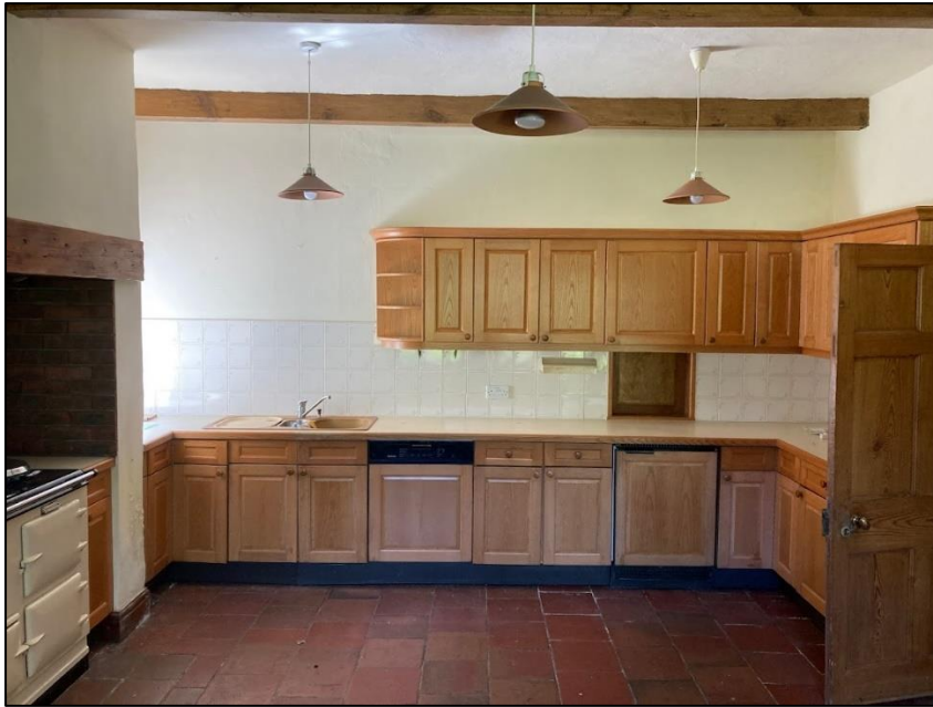
Photograph 14 showing the interior of the building
