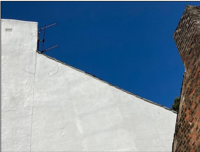
Photograph 11 showing one of the gable ends of the building
