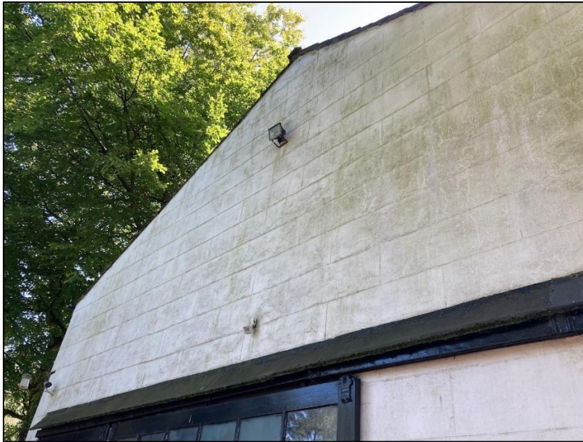
Photograph 12 showing the Garage gable end
