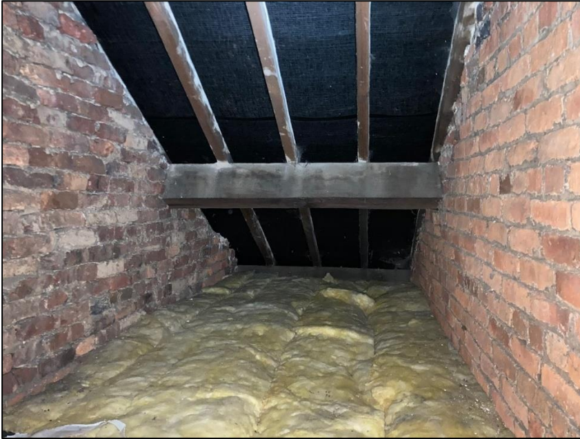
Photograph 18 showing the roof void space
