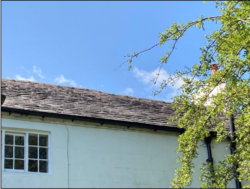
Photograph 8 showing a slate covered section of the roof
