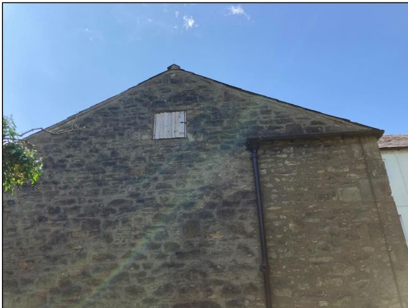
Photograph 17 showing the external access hatch to the roof void space
