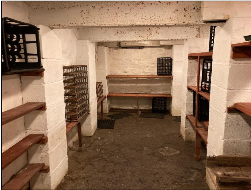
Photograph 22 showing the basement
