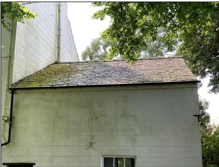
Photograph 9 showing the garage roof
