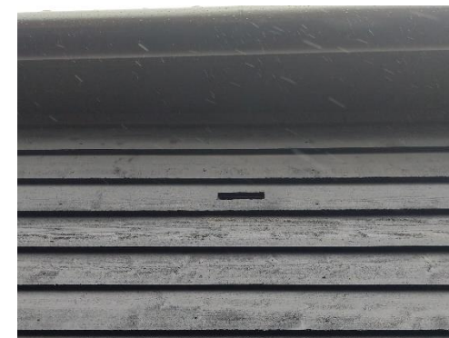
Access to the bat boxes cut into weather boarding. The holes can be cut by scalloping the underside of the board where it covered the board below to reduce water ingress
