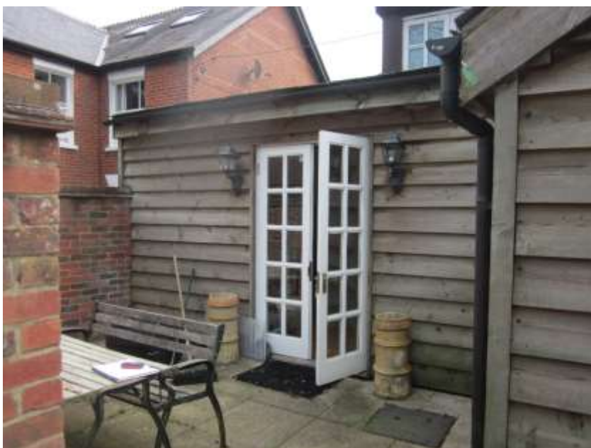
Rear Elevation showing double doors from kitchen area
