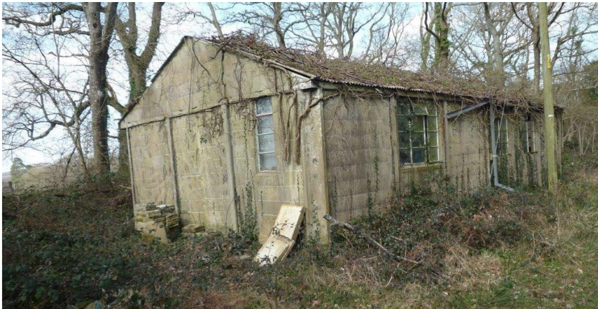
Photo 6 – Rear view of existing structure to be converted.
