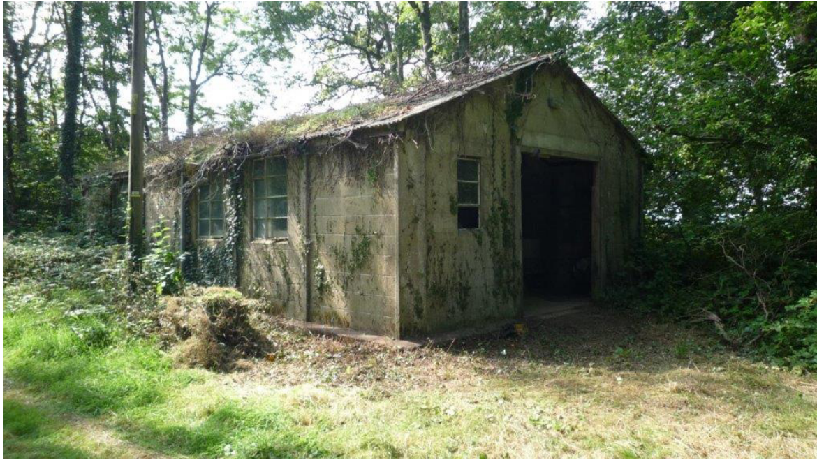
Photo 5 – Front view of existing structure to be converted.
