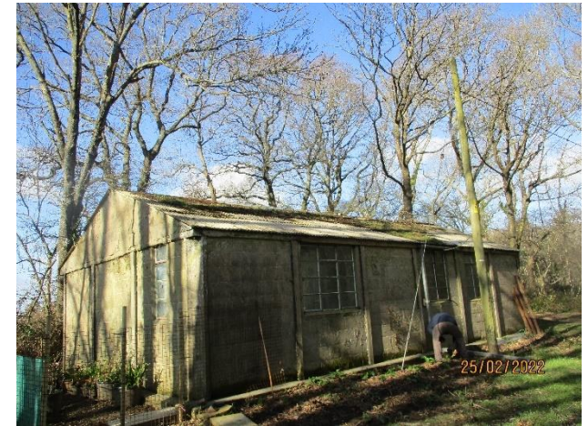
Photo 3: East and south elevations of barn.
