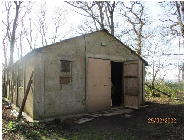
Photo 2: North elevation of barn.
