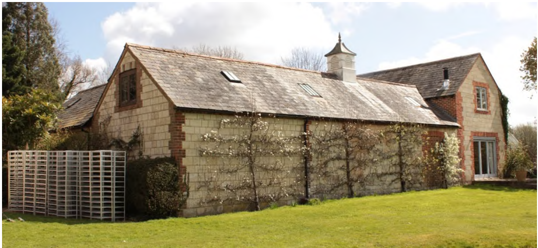
Figure 17 The historic west range of the stable, rear and north gable elevations.
