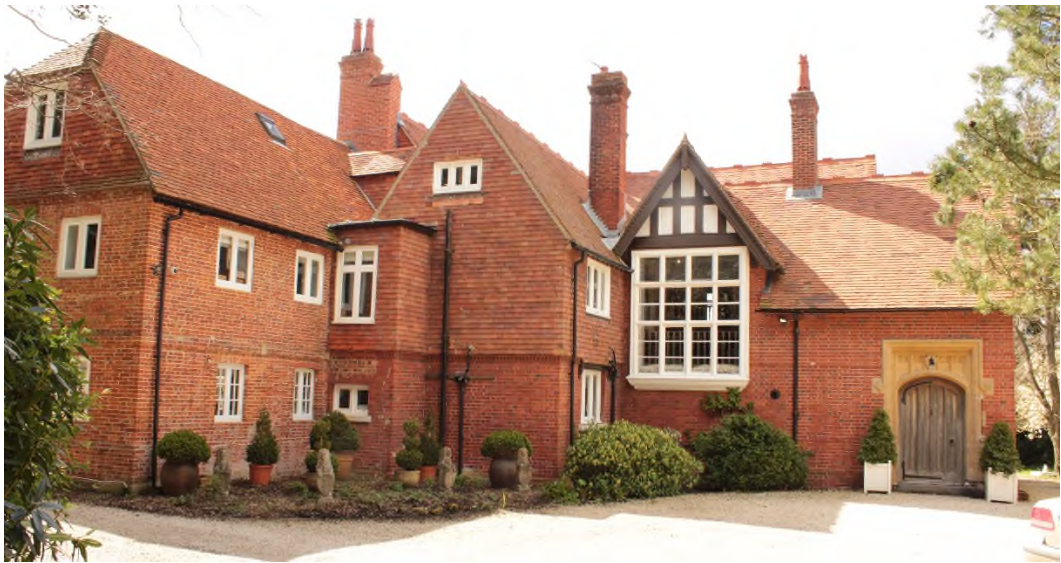
Figure 4 The entrance front to the east.
