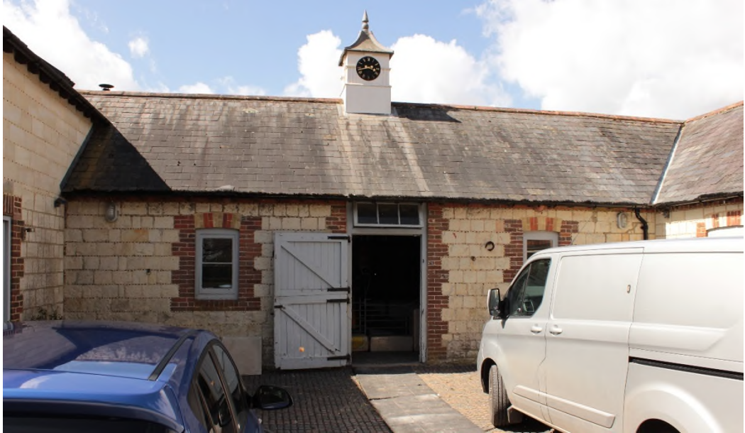
Figure 16 The east elevation of the historic stable block.
