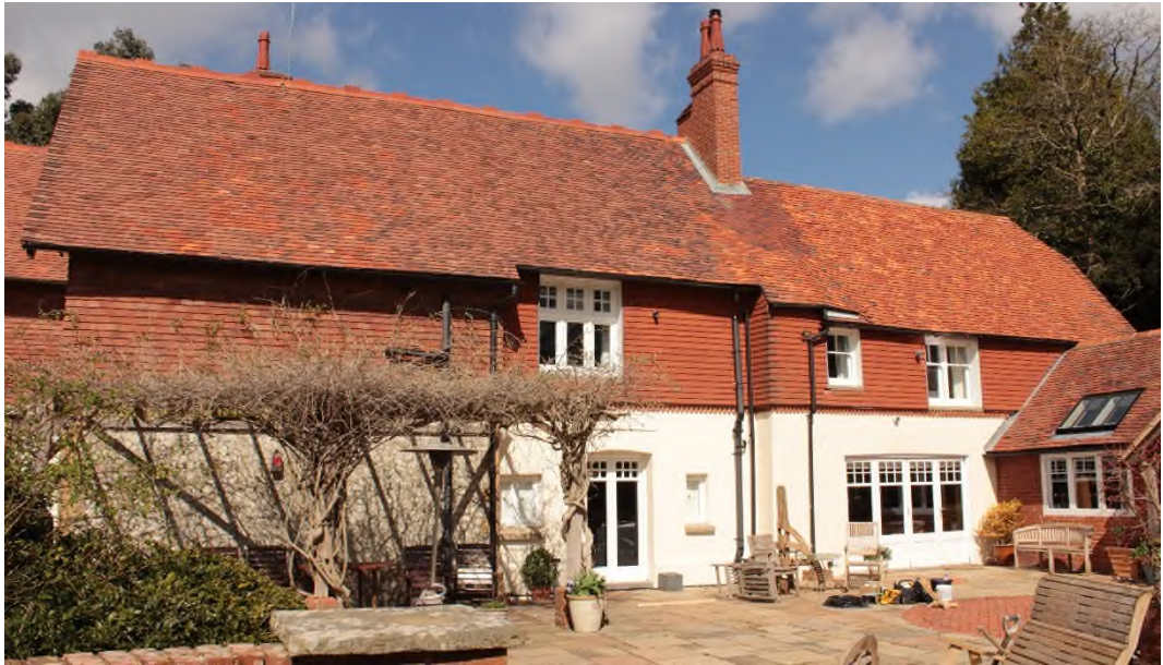
Figure 5 South elevation of the east range.
