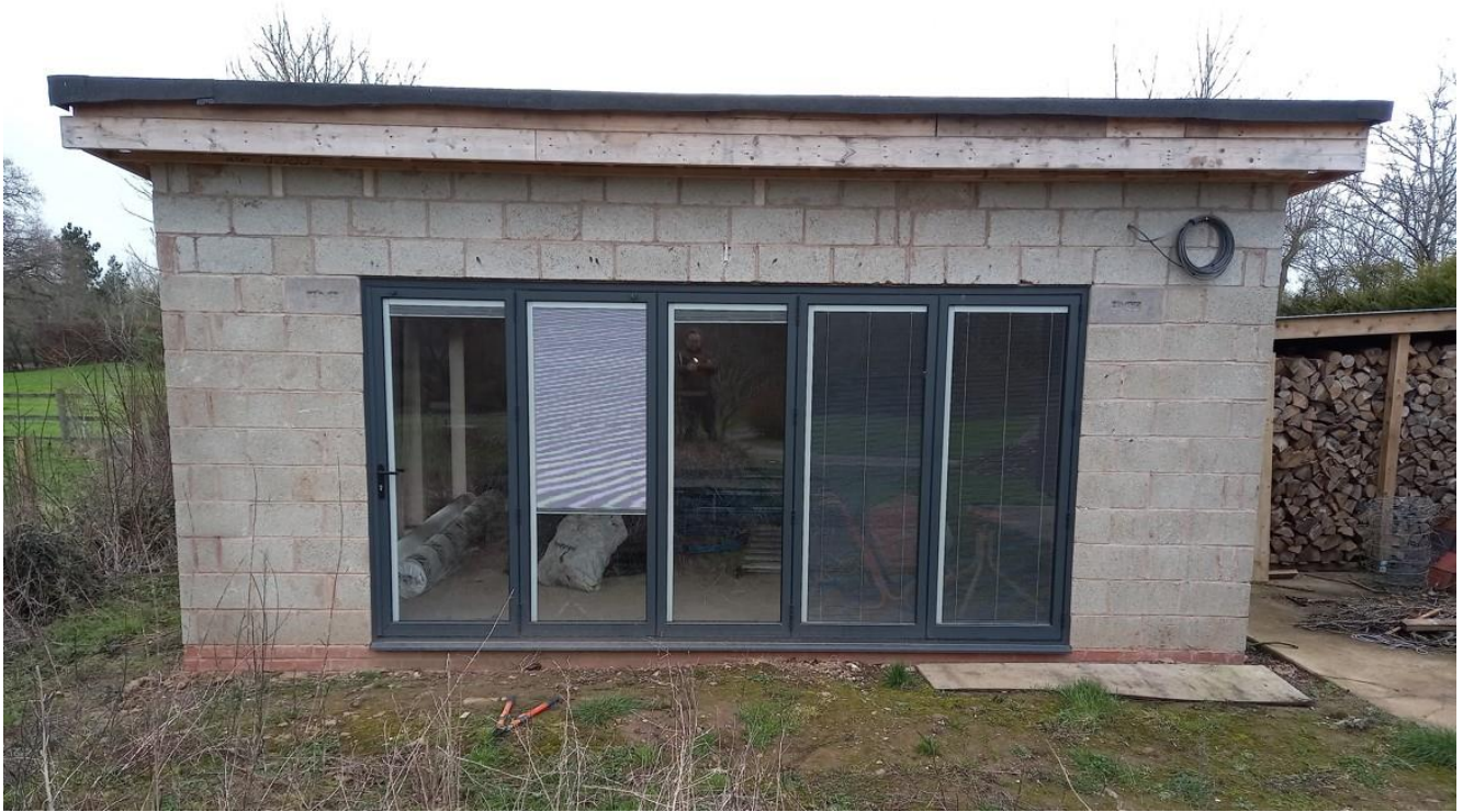
Front elevation of building 2 (facing east).
