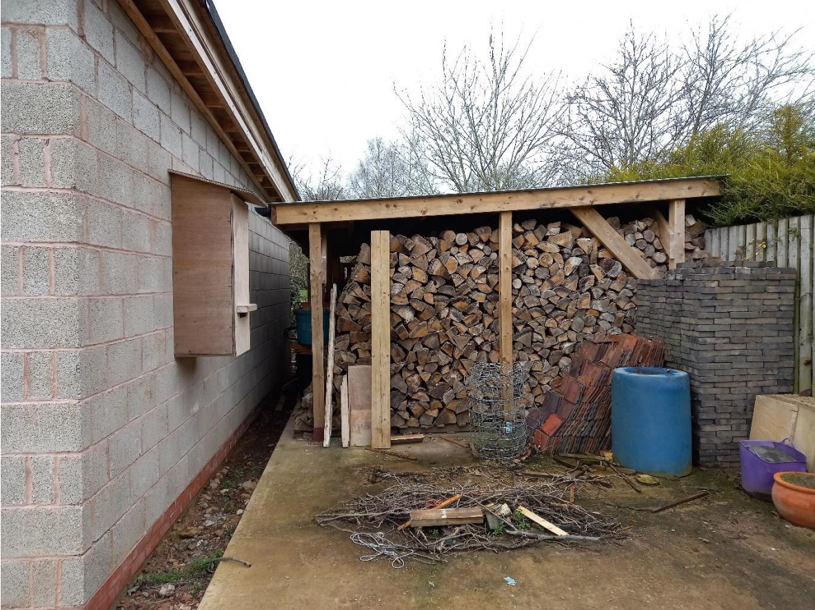
Side elevation of building and wood store (facing north).
