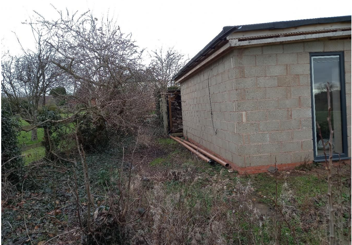
Rear elevation of building 2 (facing west).
