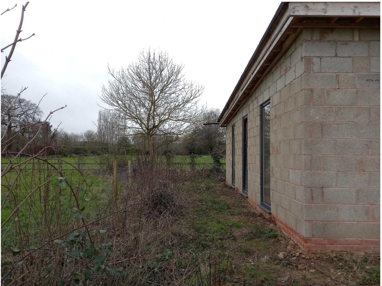
Side elevation facing field (facing south).
