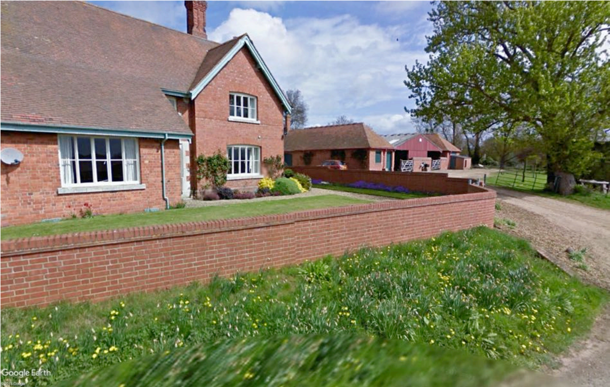
Red House Farmhouse with the buildings proposed for conversion in the background (NB. The central Dutch barn element has been removed).
