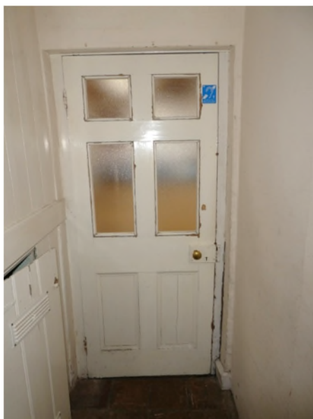
Figure 27: Part-glazed 6-panelled door on the north side of G11
