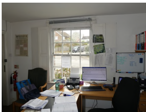
Figure 20: Sash window and internal shutters on the south side of G4
