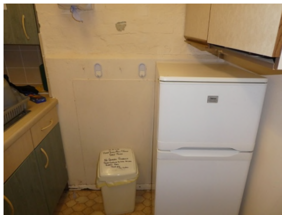
Figure 29: Chimney breast with blocked fireplace in G12
