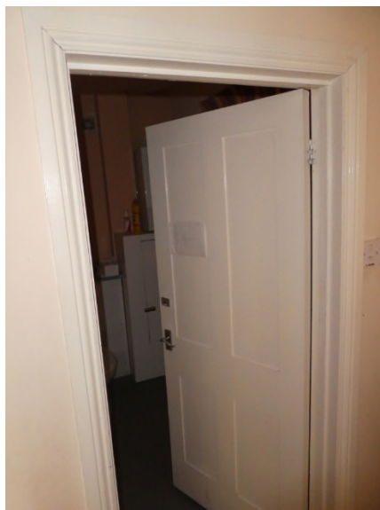
Figure 61: 4-panelled door to F8
