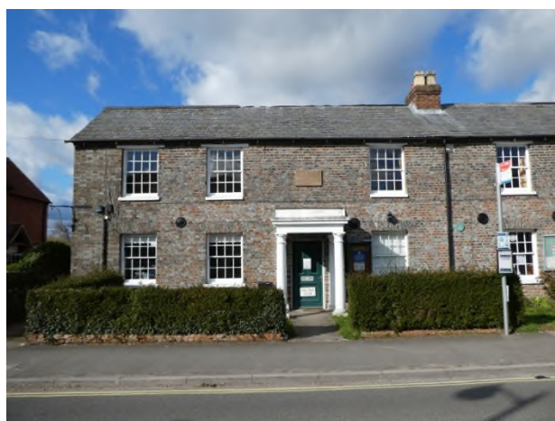
Figure 8: Brick plinth along the front boundary of 35 George Street
