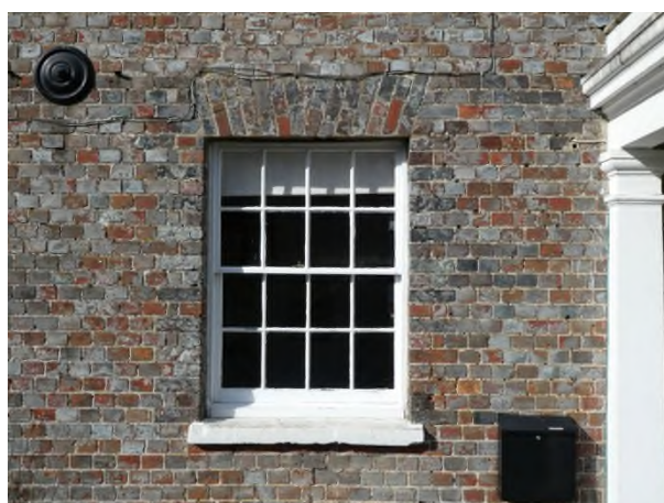
Figure 17: Phase 1 sash window opening
