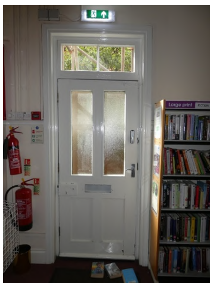
Figure 32: Part-glazed panelled door with overlight on the RHS of the west elevation of G13
