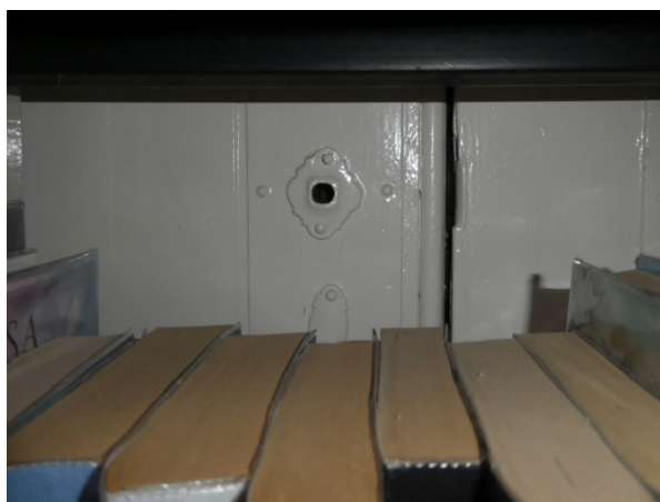
Figure 37: Cupboard doors concealed behind shelves on the east side of G13
