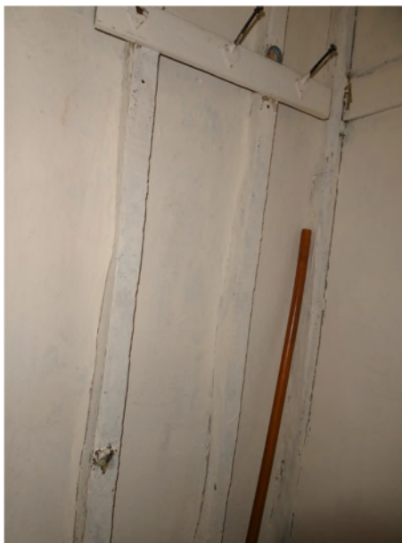
Figure 51: Stud partition in the cupboard
