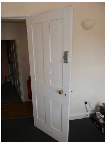
Figure 52: 4-panelled door to F3
