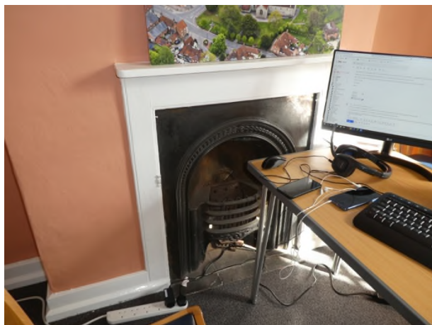
Figure 53: Wooden fire surround and arch plate register grate in F3
