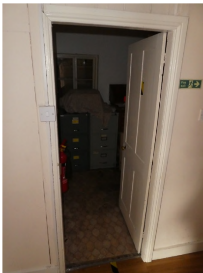
Figure 55: 4-panelled door to F5
