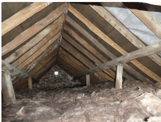
Figure 63: Phase 1 roof structure
