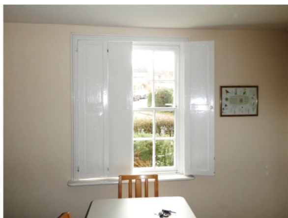
Figure 22: Sash window and panelled shutters in G6
