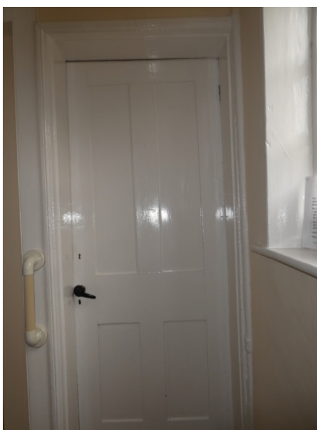
Figure 39: 4-panelled door to F1 at the top of the dog-leg staircase
