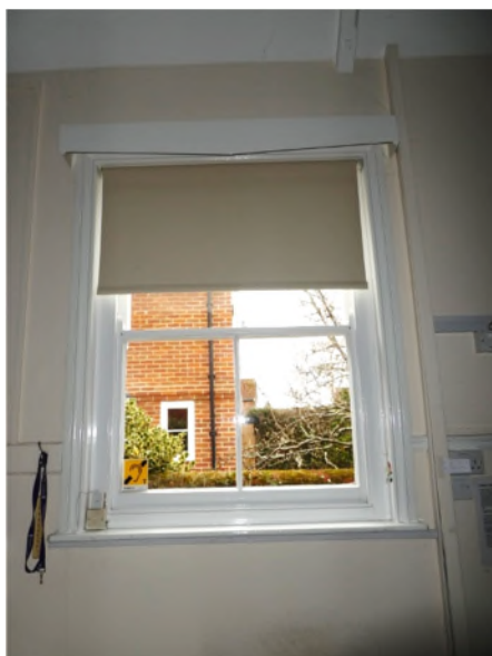
Figure 34: 2-over-2 horned sash window on the western side of G13
