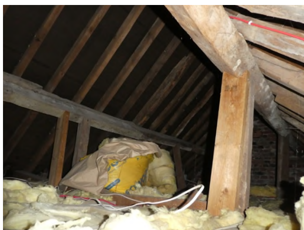
Figure 62: Phase 2 roof structure
