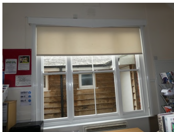
Figure 35: 2-over-2 horned sash window with side lights on the north side of G13
