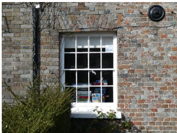
Figure 16: Phase 3 sash window opening
