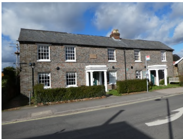
Figure 1: Front elevation of 35-37 George Street
