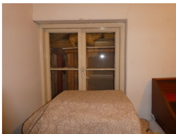
Figure 57: 2-light casement window on the north side of F5
