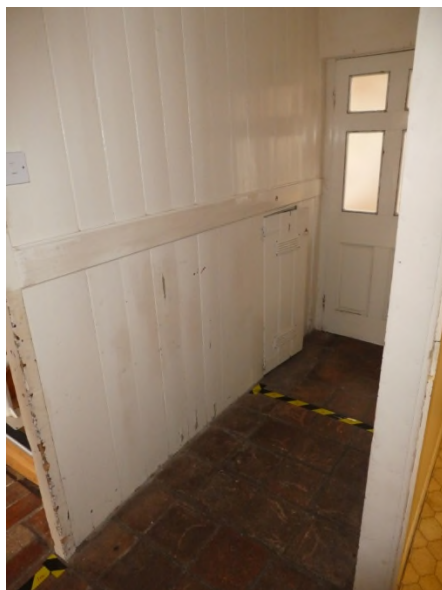
Figure 26: Matchboard panelling and plank door to the under stairs cupboard
