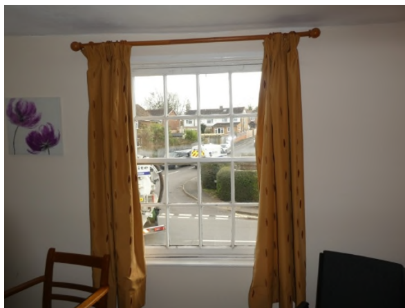
Figure 49: Sash window on the side of F2
