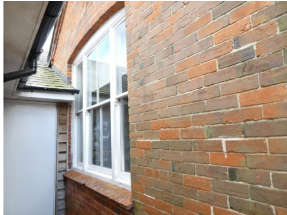
Figure 7: Part of the north elevation of Phase 4
