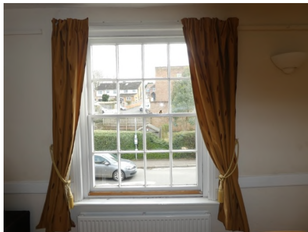
Figure 45: Central sash window in F1
