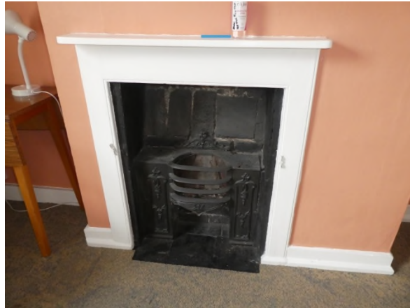
Figure 48: Wooden fire surround and hob grate
