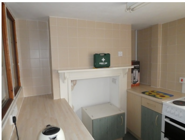
Figure 24: Chimney breast and wooden fire surround in G10
