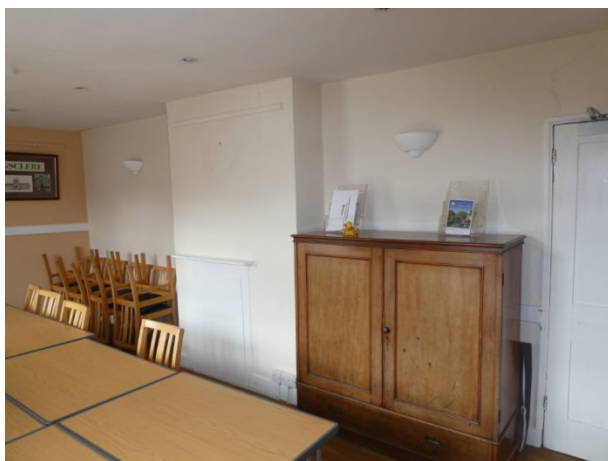
Figure 41: Chimney breast with wooden surround to a blocked fireplace in F1
