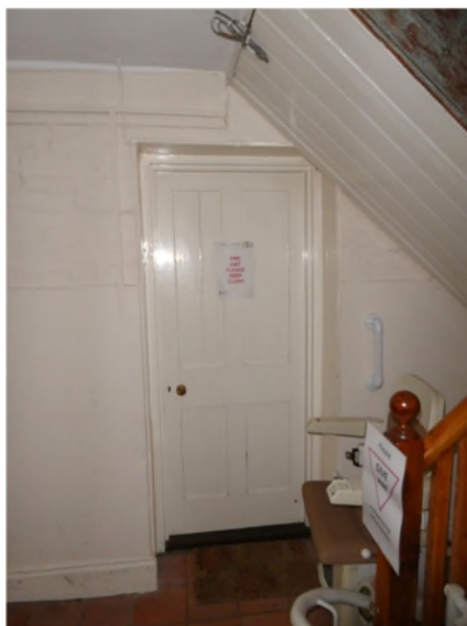
Figure 31: 4-panelled door from G11 to G13
