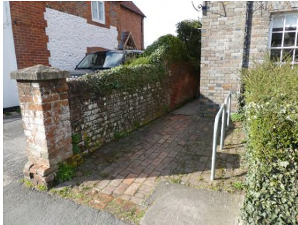
Figure 9: Western boundary wall
