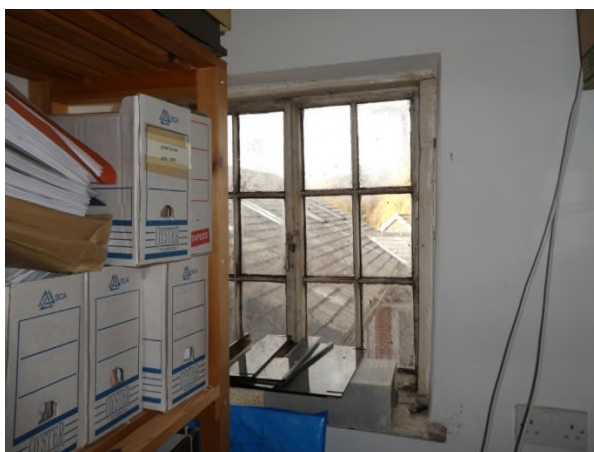
Figure 60: 2-light casement window on the north side of F7
