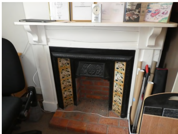
Figure 19: Wooden fire surround and late Victorian style grate in G4
