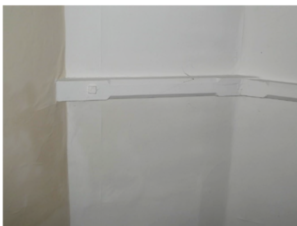
Figure 38: Detail of the roof structure in G13
