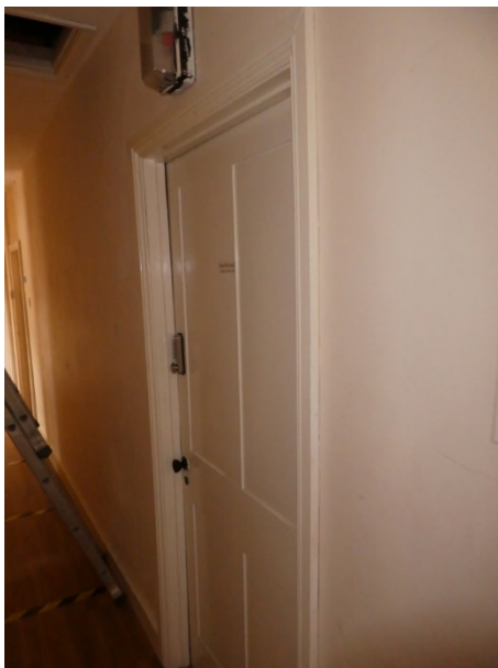
Figure 58: 4-panelled door to F6
