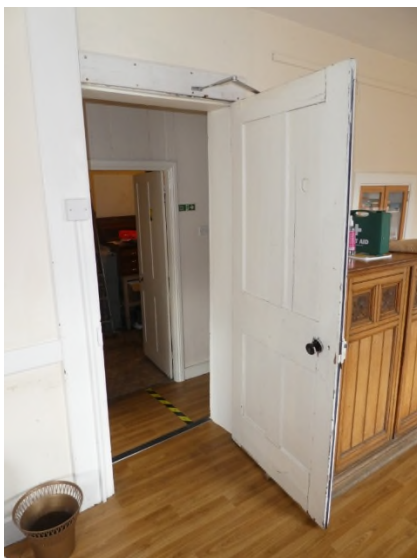
Figure 40: 4-panelled door to F1 from the landing
