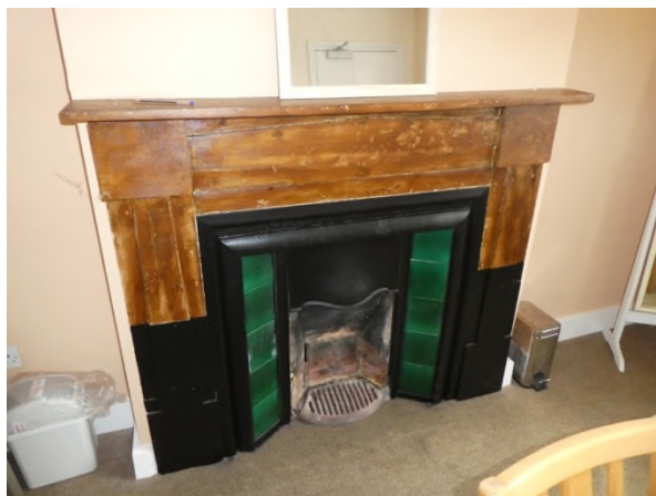
Figure 23: Wooden fire surround and cast iron grate in G6
