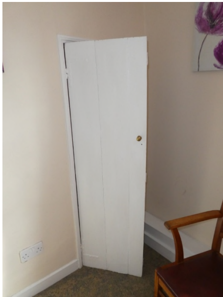
Figure 50: Plank and batten cupboard door with L-hinges
