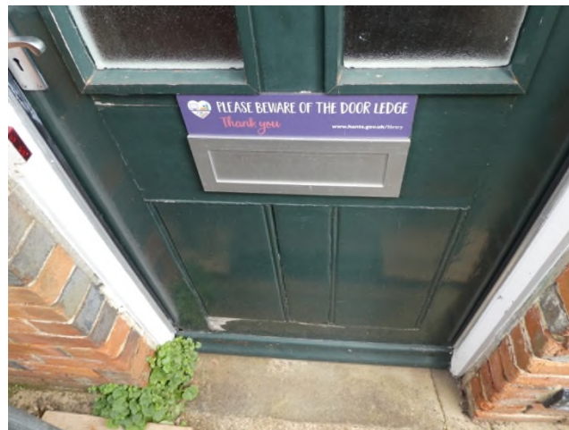
Figure 19: Detail showing the original lower panels and the modern glazed panels
