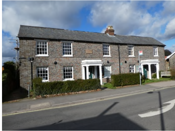
Figure 9: 19 th century 8-over-8 sash windows on the front elevation
