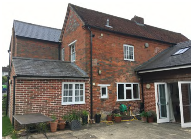
Figure 11: Mix of late 19 th -early 20 th century casements and modern casements on the rear elevation (north)
