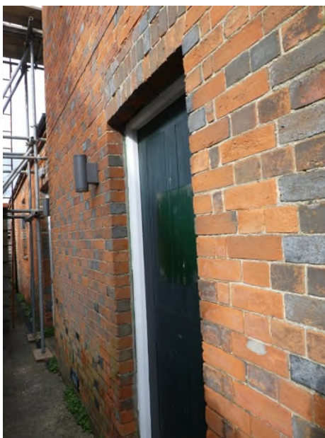
Figure 16: Panelled door on the west elevation of Phase 3
