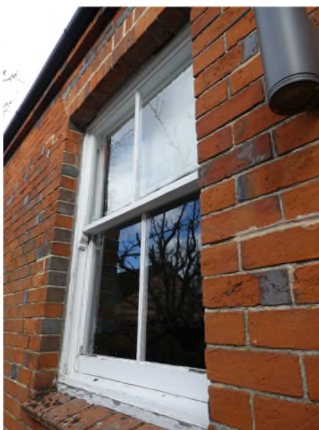
Figure 13: Late 19 th to early 20 th century sash window on the west elevation (library rear wing)
