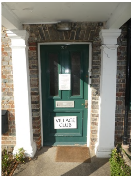
Figure 14: Modern replacement door at No. 35
