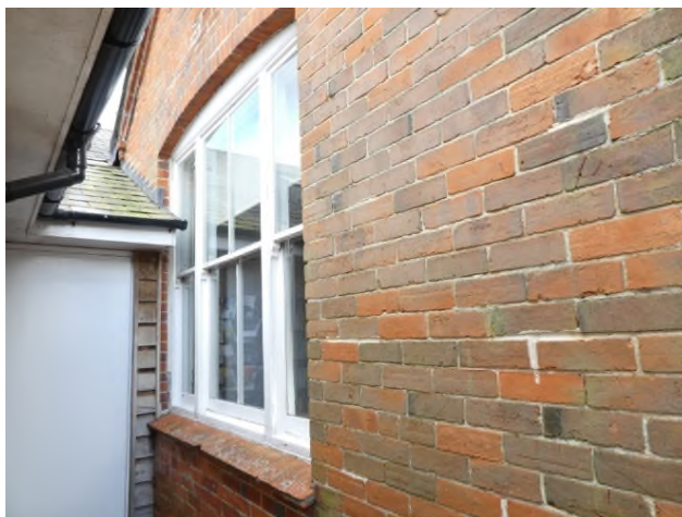
Figure 12: Late 19 th to early 20 th century tripartite sash window on the north elevation of the rear library wing
