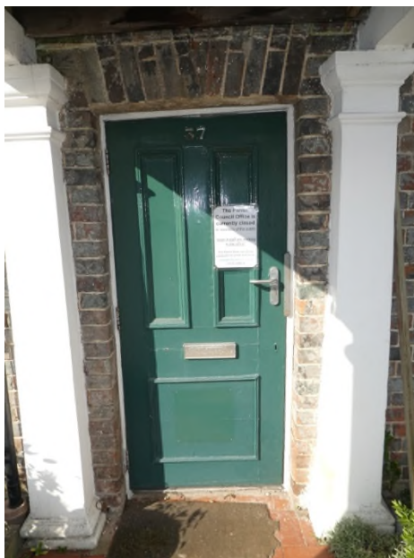
Figure 15: Front door at No. 37
