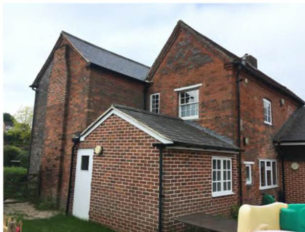
Figure 10: 20 th century sash and fixed light on the east elevation
