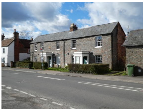
Figure 1: Front elevation of 35-37 George Street
