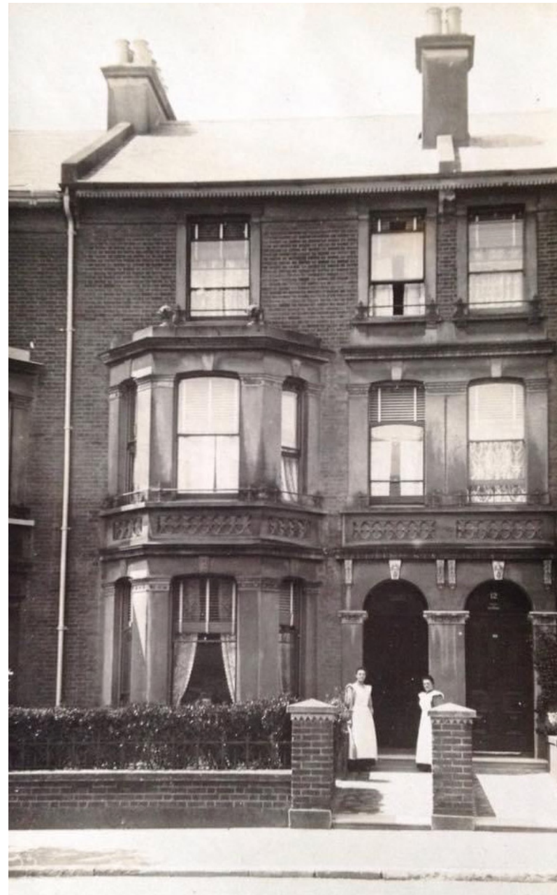
existing archive photograph of number 11 Westbourne Villas
