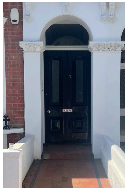
original door style present at 13 Westbourne Villas
