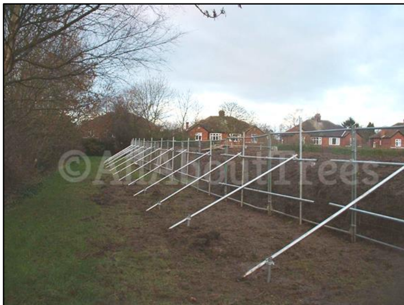
Figure 2 - Actual barrier erected on site
