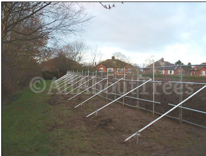
Figure 3 – An example of a barrier erected on a site
