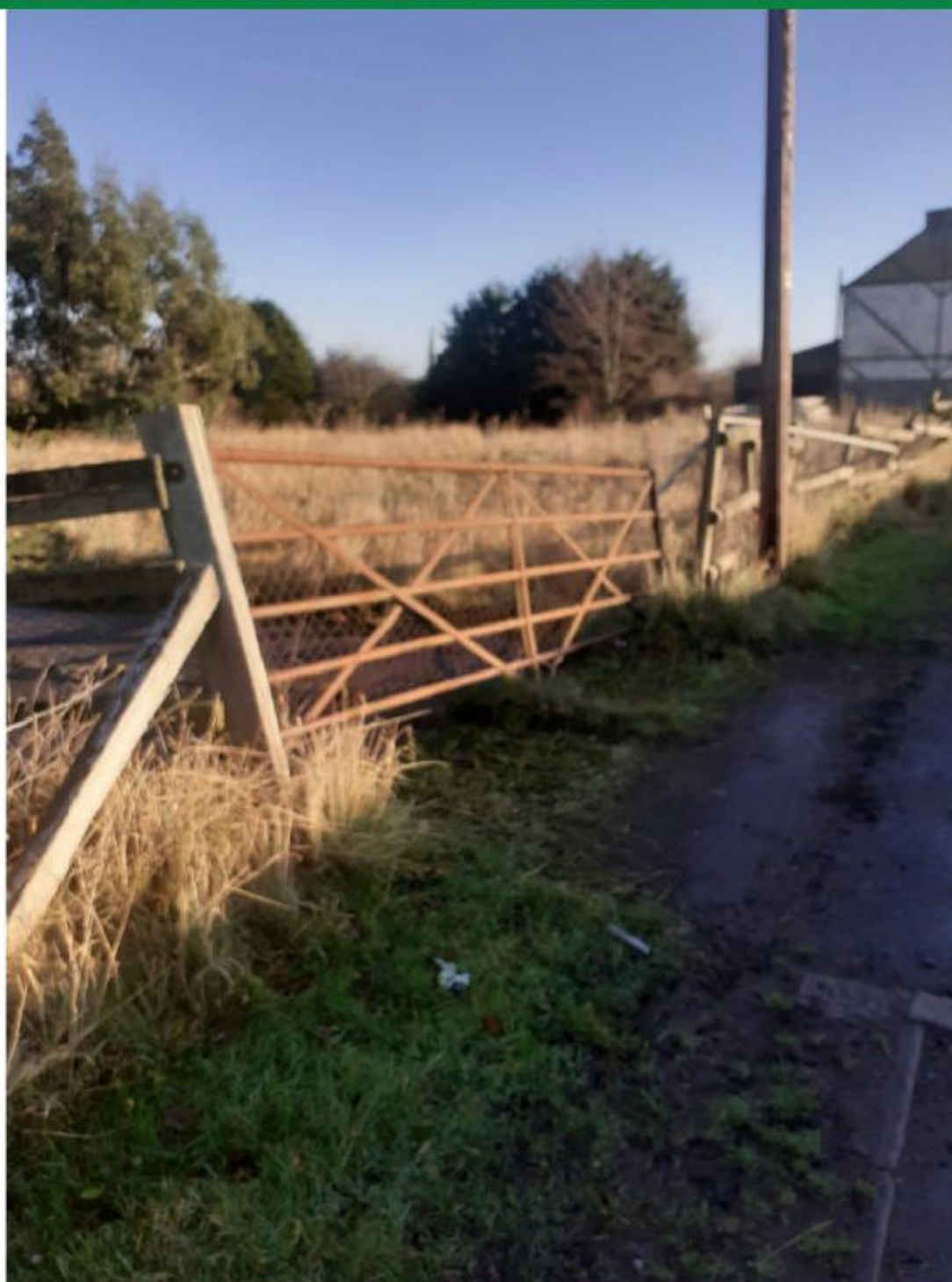
PLATE 2 – ACCESS GATE AT THE CENTRE OF THE SOUTHERN BOUNDARY
