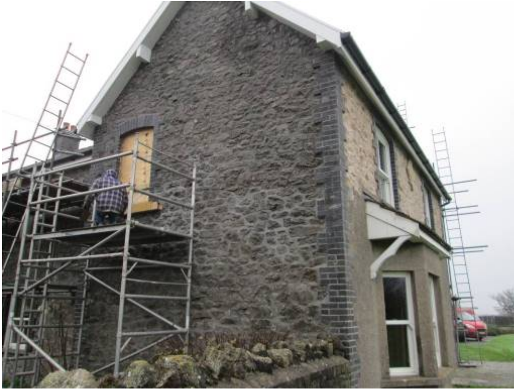
Picture ref 04 – Rear West Elevation as Existing – walls being repointed (November 2020).
