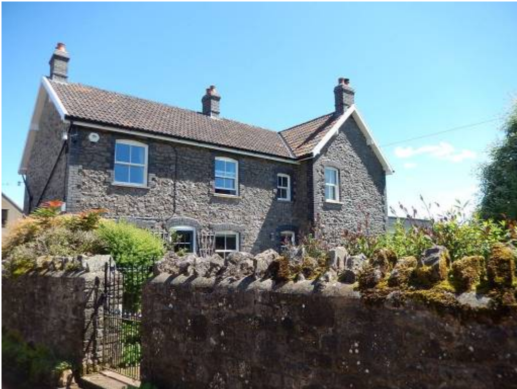
Picture 07 – Rear West Elevation as Built and viewed from Ash Lane (June 2022)
