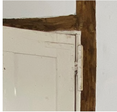
L-h-hinge came into use in the late 17th century, plain ones as here are the norm throughout the 18th century and into the early 19th century.
