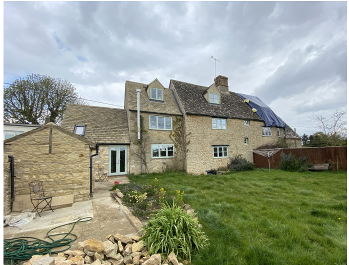
Rear elevation with small modern outbuilding on the left. This elevation has been heavily altered with dormers added and larger glazed windows and doors in the extension.
