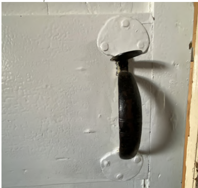
Round ended upright door handles are the simplest form of latch operated handles and mostly date from the 18th century when the ends can be quite large as here. Earlier versions from the 17th century are slightly smaller and often have leaf shaped decorated ends.
