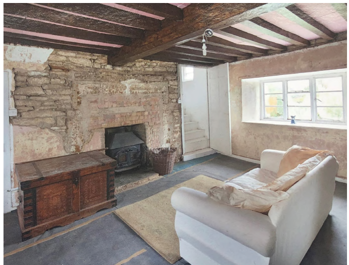
Exposed walls 2014 show the progressive infilling of the fireplace with a mix of brick and stone blockwork.
