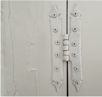
H-hinge very common in the late 17th century and the early 18th century and usually used for lighter internal doors and cupboard doors. During the course of the 18th century the decorative ends are often lost and the plain H-hinge becomes the ubiquitous form in use.
