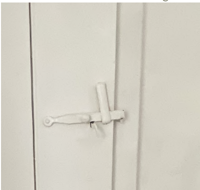
The small round knob on the latch reveals that this is a much later fixing from the mid-19th century.
