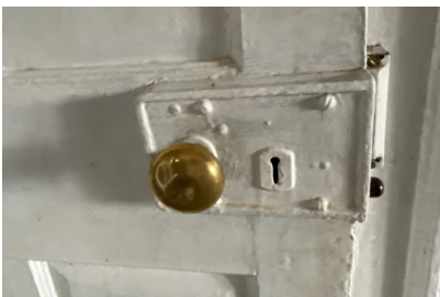
Brass lock cases became popular in the 18th century incorporating lock, latch, and handle in one unit. Its' use on an internal door indicates increased interest in security perhaps as a result of several families sharing an interconnected space.
