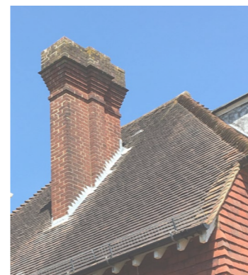
Reference Point Corbelled brickwork of the existing prominent chimney
