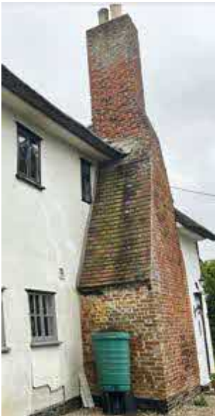
Figure 8: Concrete Verge to Chimney Stack and Extract
