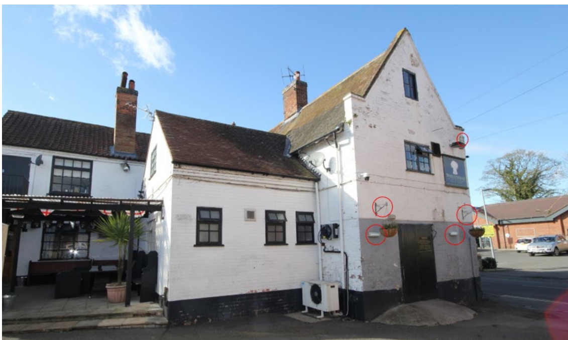
Plate 20: The fixtures to be removed from the west elevation.
