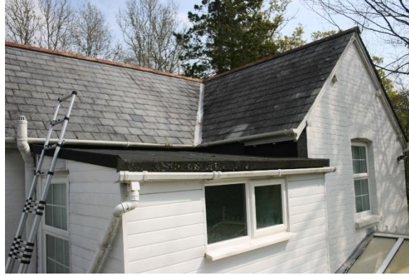
Photo 7: Gaps in dormer fascia on western elevation. Photo 8: 1st floor uPVC extension.
