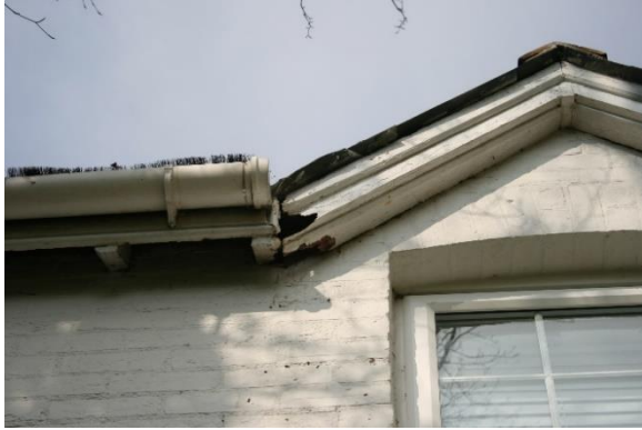
Photo 7: Gaps in dormer fascia on western elevation. Photo 8: 1st floor uPVC extension.
