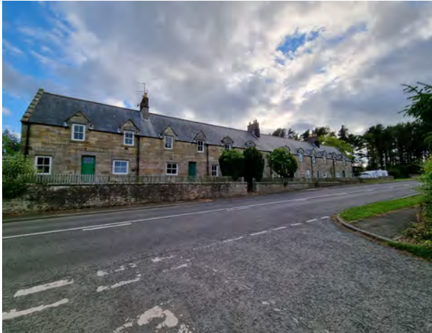
Figure 13 View of terrace, looking west/north-west
