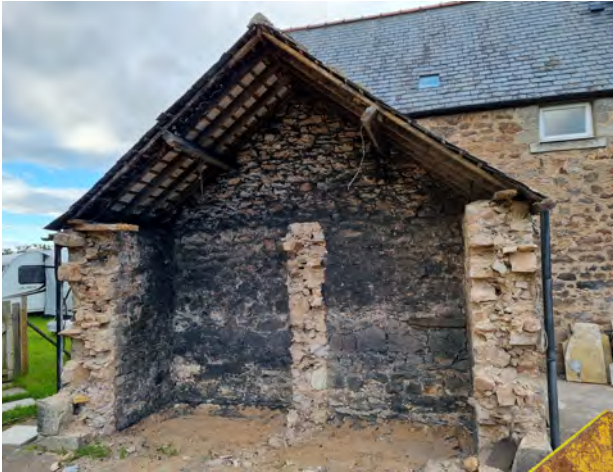
Figure 12 Gable end of rear extension
