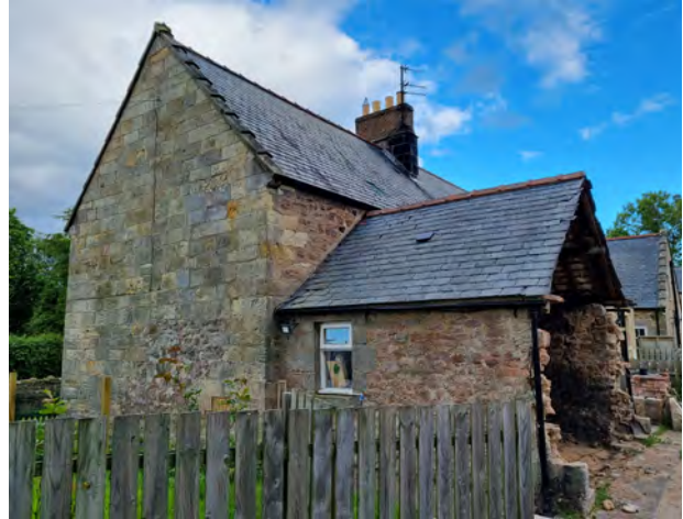
Figure 5 View of gable elevation and rear extension
