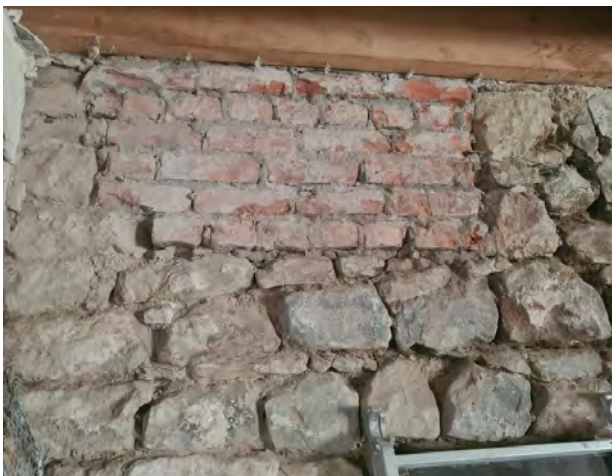
Figure 8 Interior detail of blocked window (bottom) (supplied by client)
