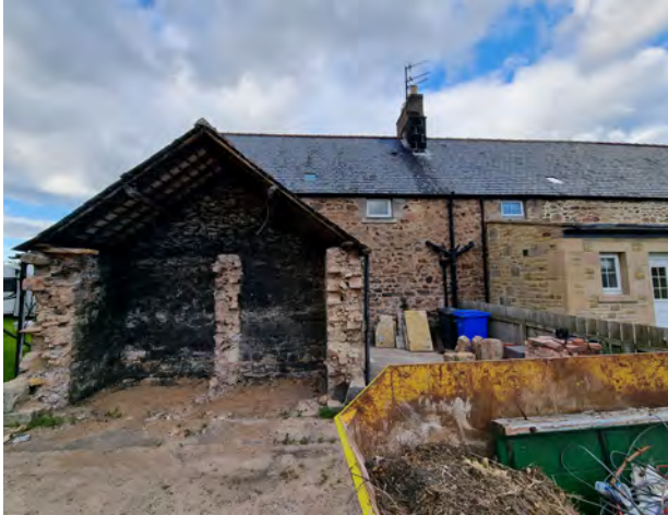
Figure 11 Rear elevation, facing east
