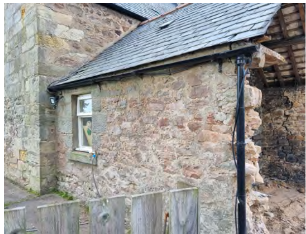
Figure 9 View of rear extension
