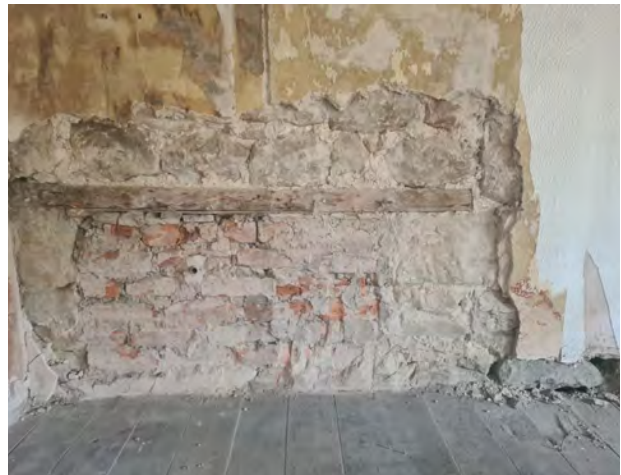
Figure 7 Interior detail of blocked window (top) (supplied by client)
