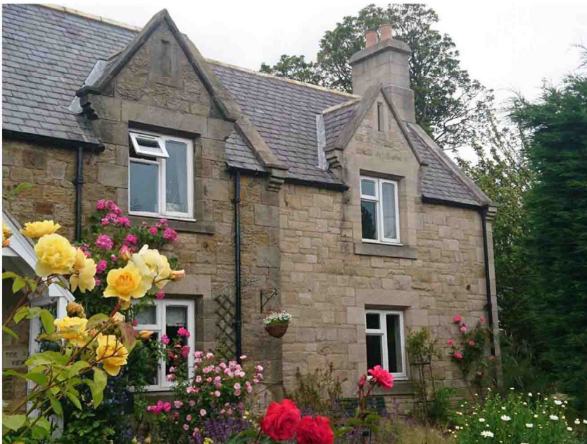
Cottage Extension 3 in Lesbury
