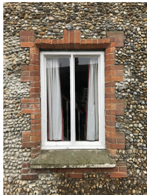
Details on the original Gate Lodge building
