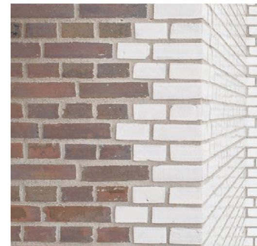
Glazed brick quoins
