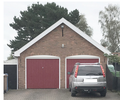
03 Poor Quality Outbuilding Nearby
