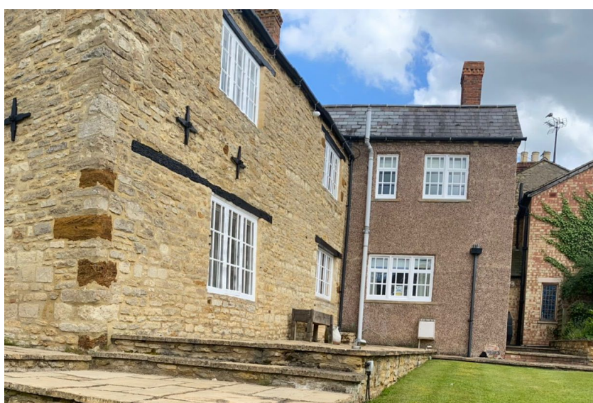
View of current cement-based pebbledash render on Victorian wing
