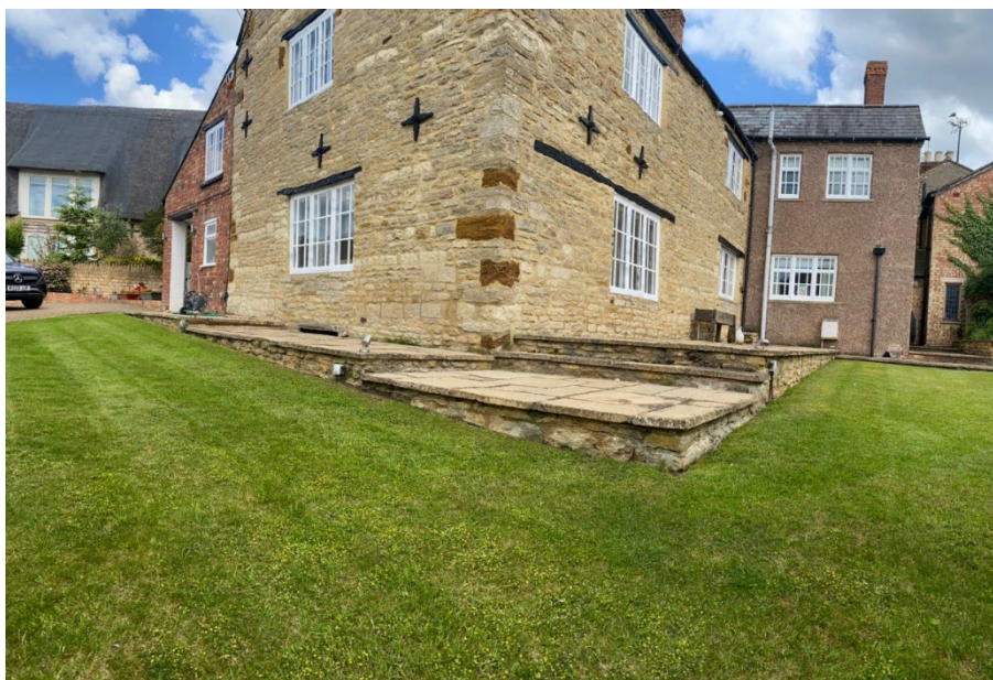
Photograph showing the elevated concrete-paved patio to the south and west elevation to be removed and reinstated to grass, with a 900mm wide ground-level path around the perimeter of the property.
