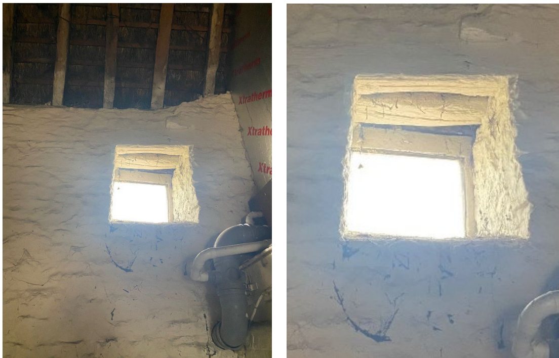
Internal view of the high-level window within the wood store
