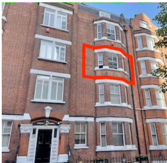
BAY WINDOW (No.s 1, 2 + 3) SEEN FROM STREET LEVEL
