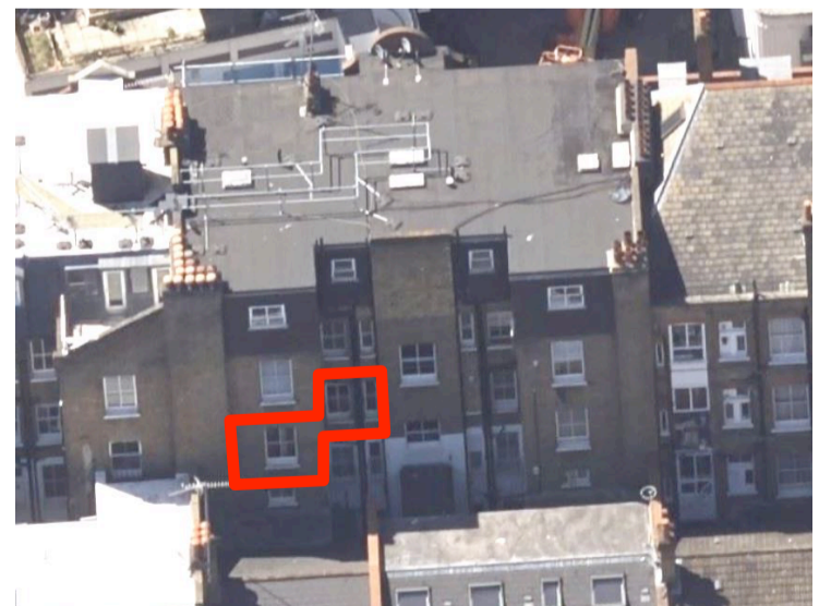
AERIAL VIEW OF REAR WINDOWS (No.s 4, 5 + 6)
