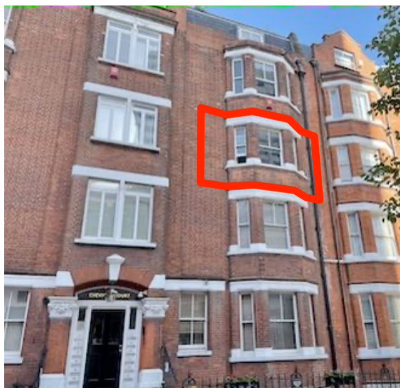
BAY WINDOW (No.s 1, 2 + 3) SEEN FROM STREET LEVEL
