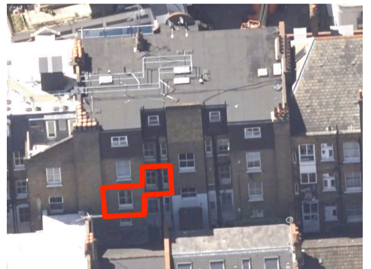
AERIAL VIEW OF REAR WINDOWS (No.s 4, 5 + 6)
