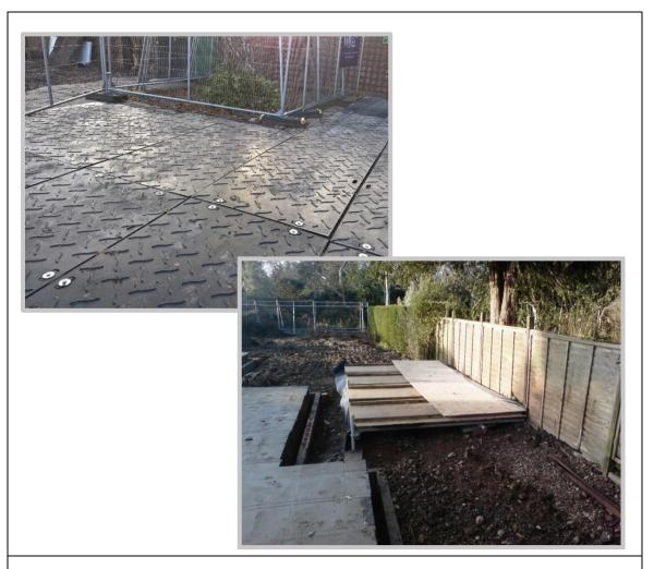
New temporary ground protection should be capable of supporting any traffic entering or using the site without being distorted or causing compaction of underlying soil.
