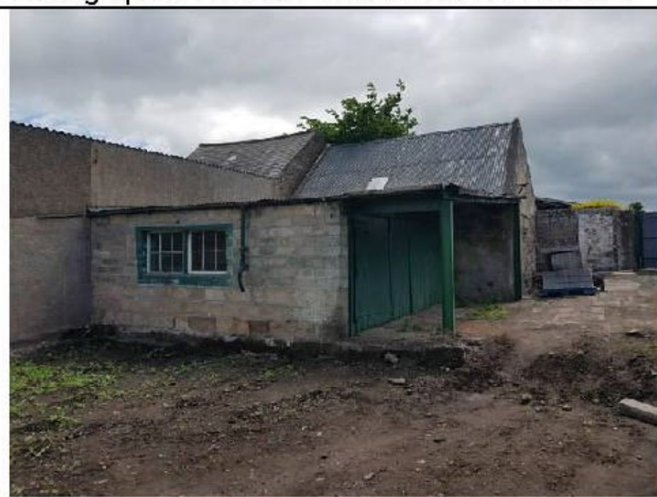
Photograph 10. Buildings at rear of garden which will be unaffected
