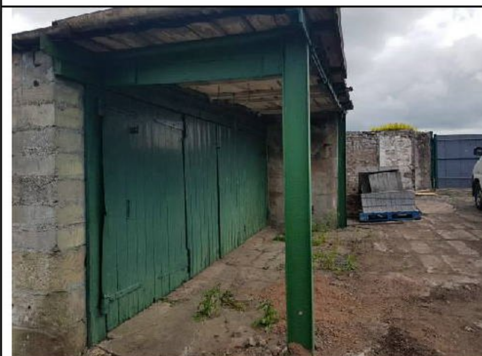
Photograph 11. Buildings at rear of garden which will be unaffected (2)
