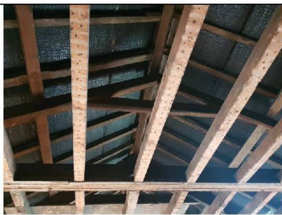
Photograph 20. Example roof construction and former void space
