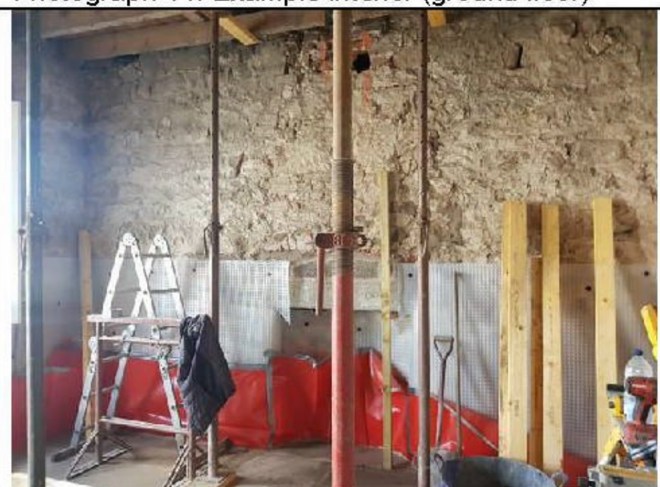
Photograph 16. Example interior (ground floor)
