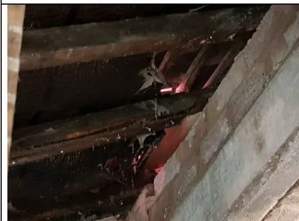
Photograph 21. Example interior access through roof coverings to exterior
