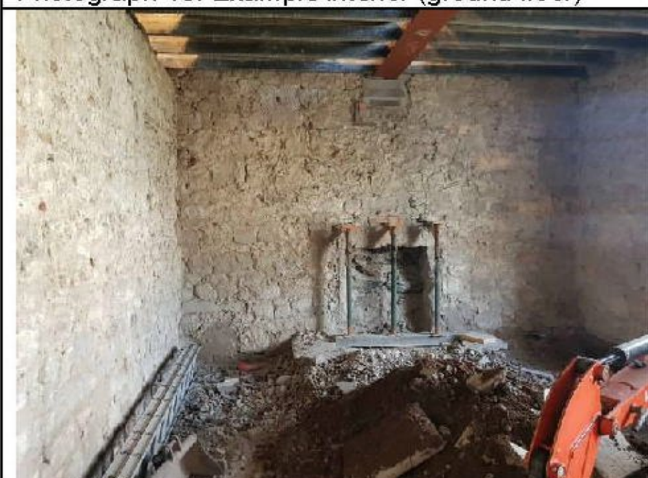
Photograph 15. Example interior (ground floor)
