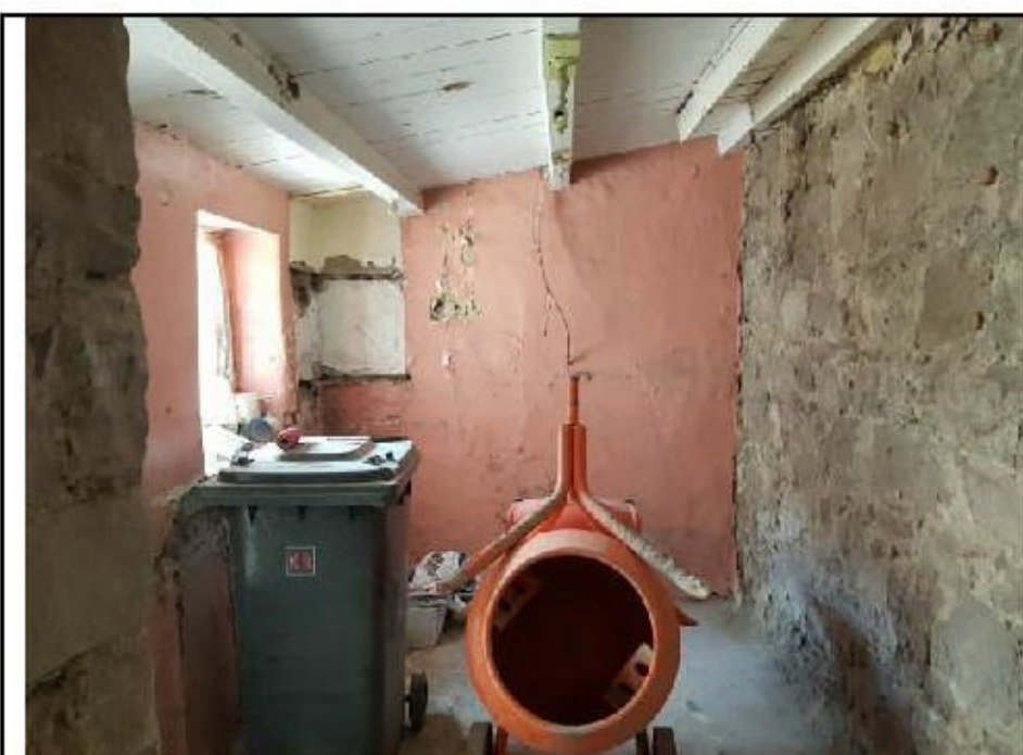
Photograph 13. Example interior (ground floor)
