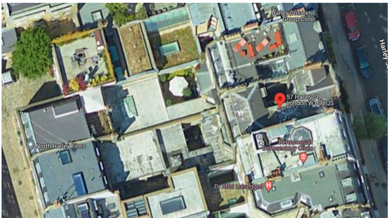
Aerial view showing roofs and lightwells to 57 and 59 Harley Street
