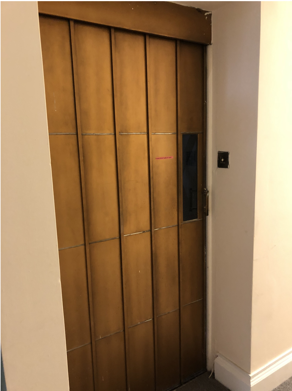
Typical Lift entrance door
