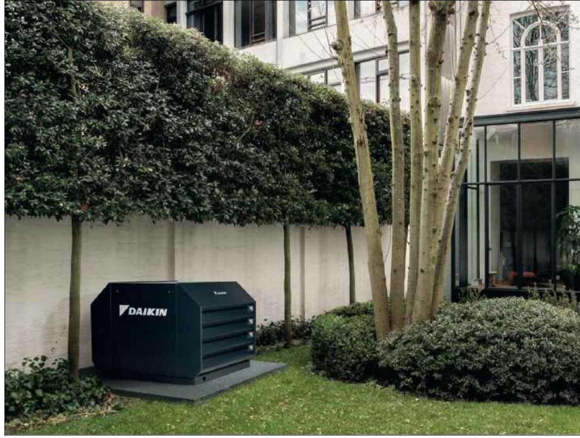
Proposed acoustic enclosure by Daikin
