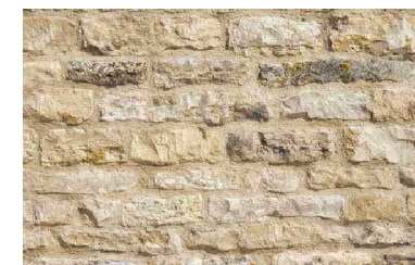
Cotswold stone walling
