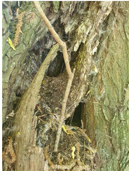
Figure 5: Cavities and decay at base on north side of stem
