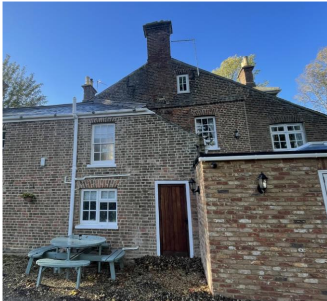
9. Change of small window to door on rear elevation.
