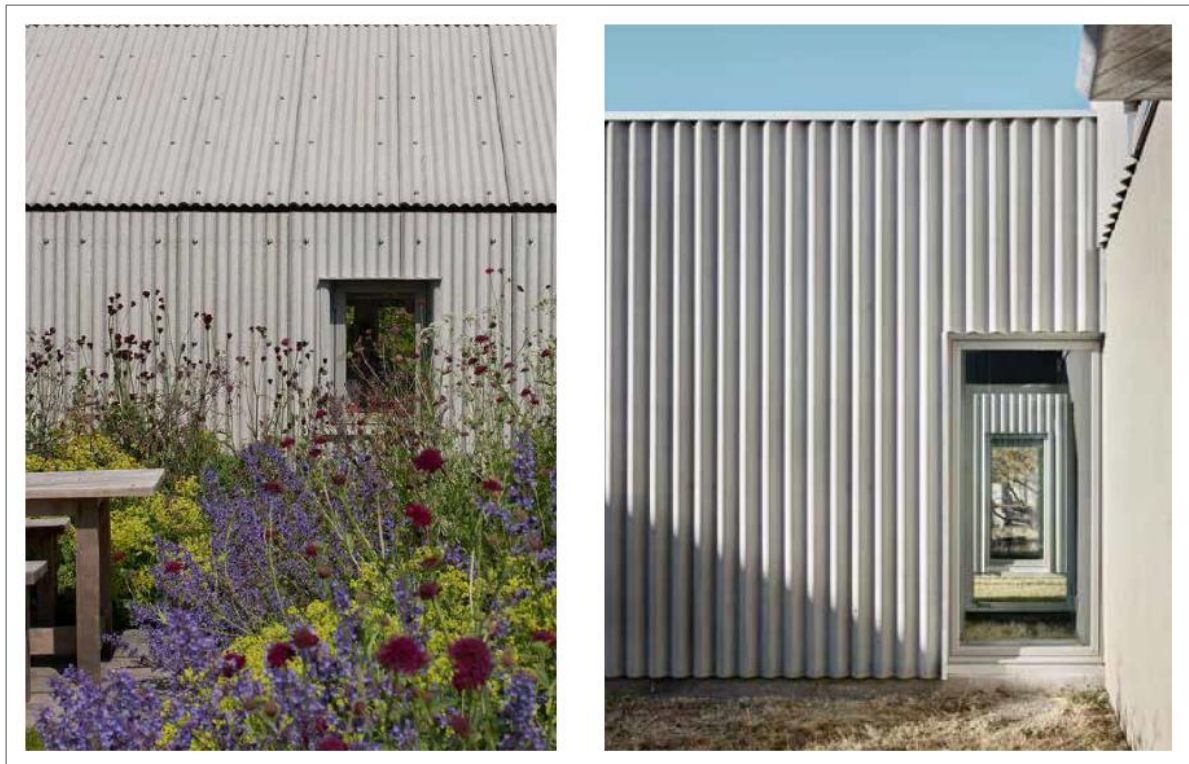
Images 11 & 12 – Illustrations of the cement fibre cladding.
