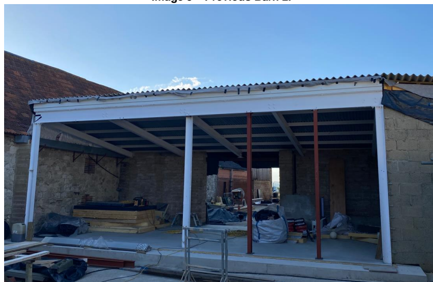
Image 6 – Barn 2 under conversion.
