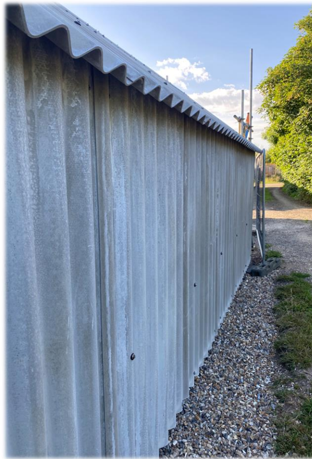
Image 13 – Cladding in-situ on Barn 1.
