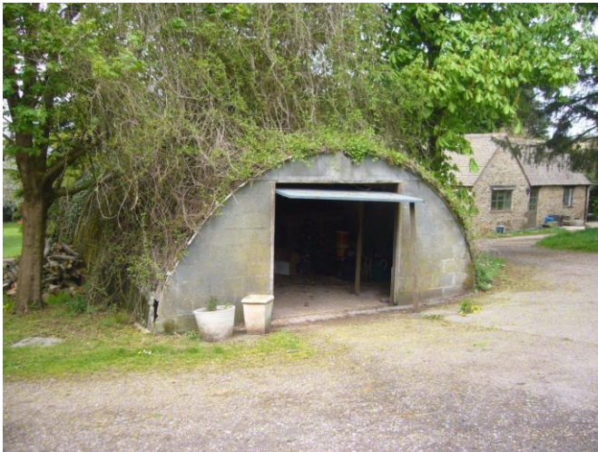
Figure 4: Building which now houses all landscaping/maintenance devices
