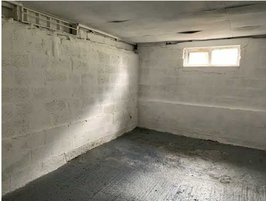
PLATE E -- EXTERNAL AND INTERNAL WALLS
