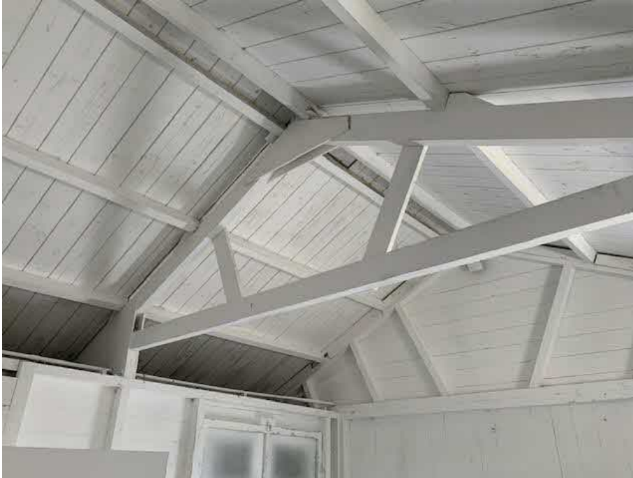
PLATE C -- ROOF STRUCTURE OF FABRICATED TIMBER TRUSSES
