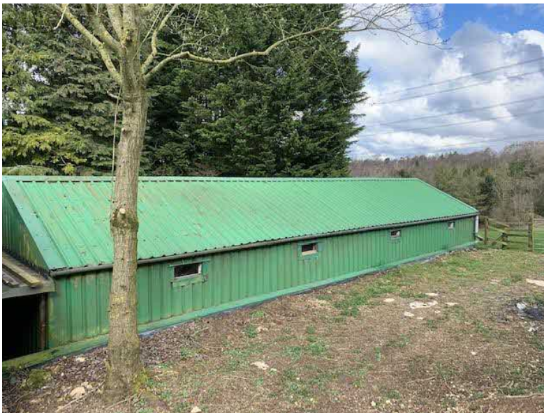
PLATE B -- GENERAL VIEW FROM EAST
