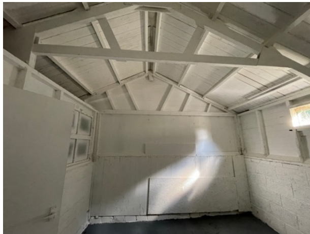
Photograph 20: Section D interior with timber sarking boards lining the roof.
