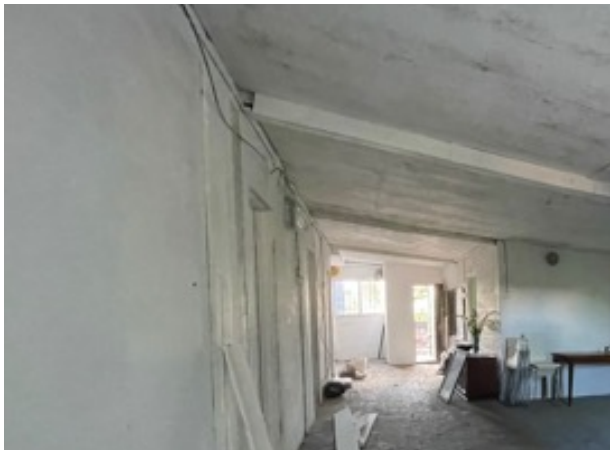
Photograph 17: View of Section C interior.
