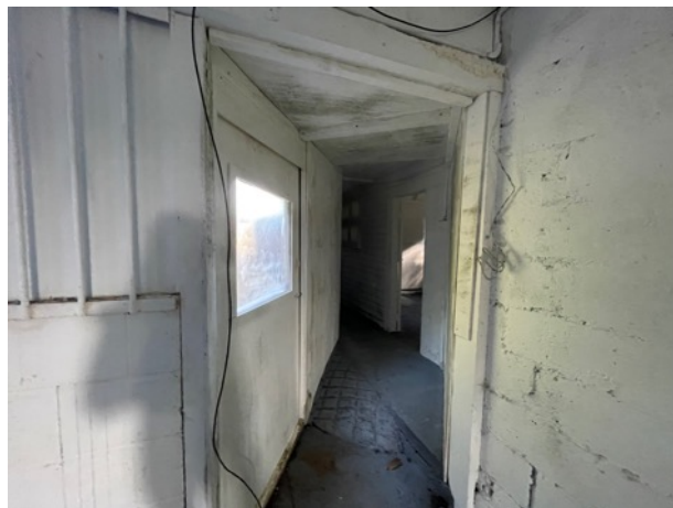
Photograph 18: Section E walkway interior joining Sections C and D.
