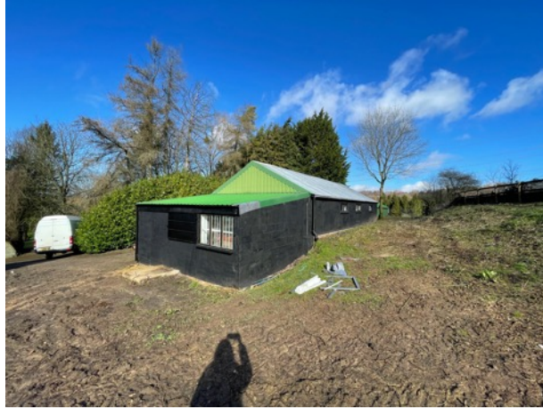
Photograph 1: General view of the building on site.
