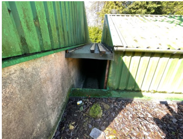
Photograph 12: Porch area between Sections B and D.
