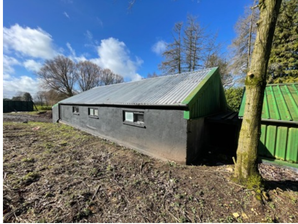
Photograph 10: East elevation of Section B.
