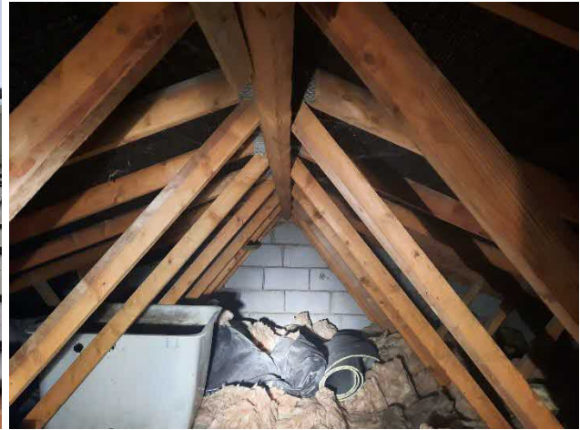
Plate 4: Loft space, looking to northeast gable.
