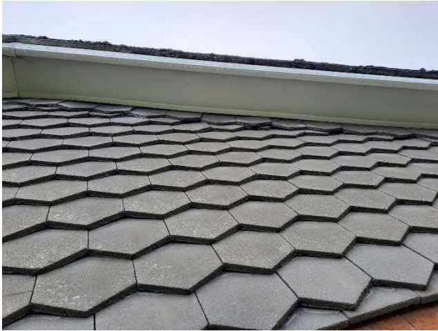
Plate 3: Hanging tiles on northeast gable.
