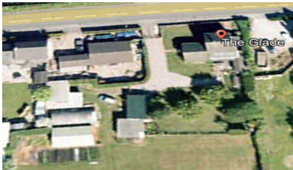
Figure 1: Shows the site in its original state in 2010.
