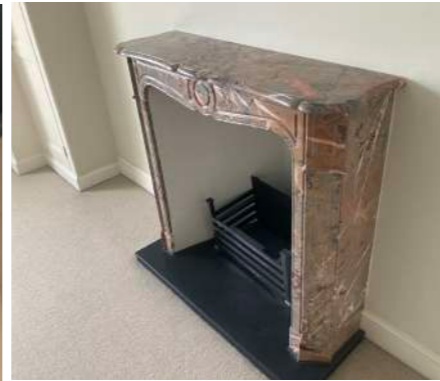
Figure 50: Existing Master Bed fire surround.
