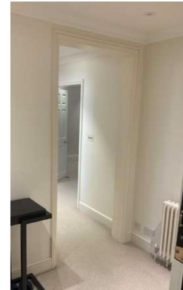
Figure 22: Existing Photo of nib walls between Entrance Hallway and Hallway.
