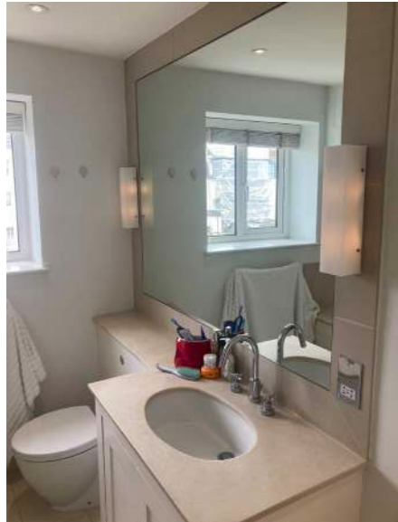
Figure 40: Existing modern fit-out & finishes in Master Bathroom.
