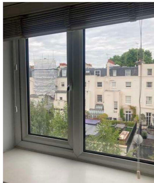
Figure 06: Existing Master Bathroom PVC double glazed casement window.
