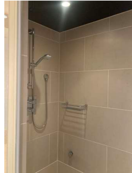
Figure 42: Existing modern fit-out & finishes in Bathroom 2.
