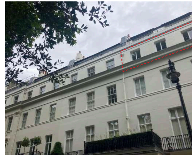
Figure 14: Looking to the left of Flat H front elevation to neighbouring properties. The casement windows to Flat H are highlighted in red.
