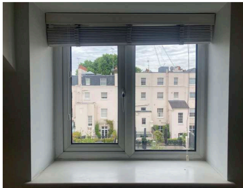
Figure 05: Existing Master Bathroom PVC double glazed casement window.
