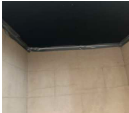
Figure 49: Existing Living Room top of chamber blocked up.
