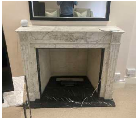
Figure 48: Existing Living Room fire surround.
