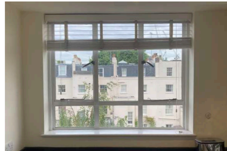
Figure 07: Existing Kitchen rear casement window.
