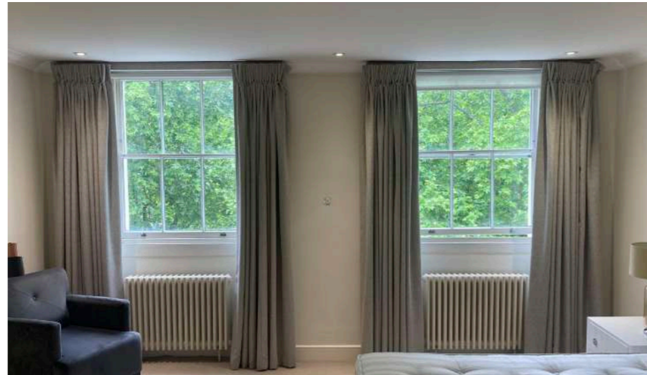
Figure 12: Existing traditional hardwood sash windows.
