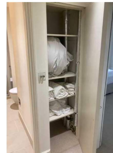
Figure 34: Existing drainage and plumbing within cupboard next to Bathroom 2.
