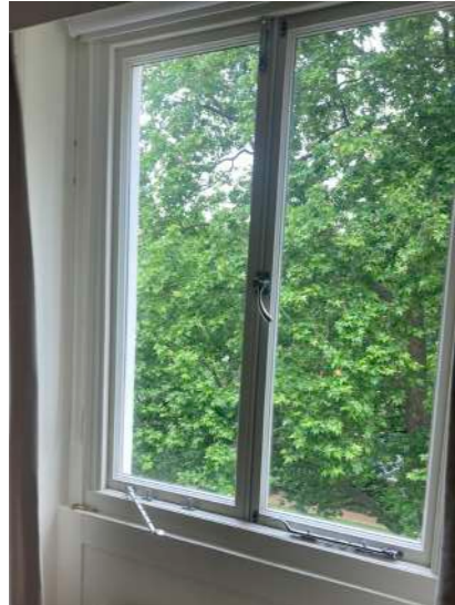
Figure 11: Existing modern panel casement window.
