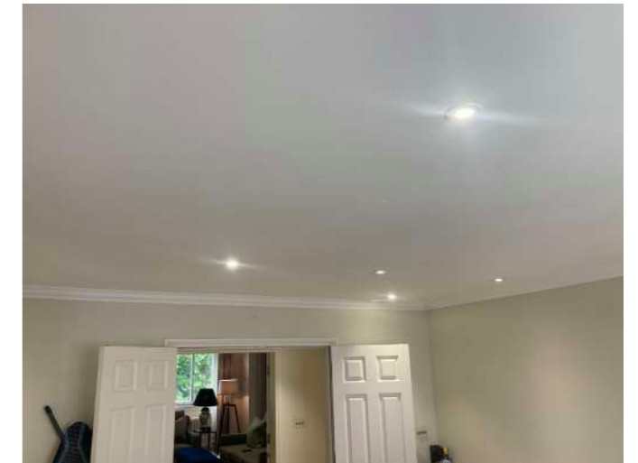
Figure 57: Existing lighting to ceiling in Dining Room.
