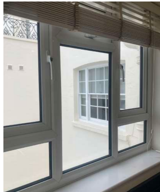
Figure 04: Existing Kitchen side elevation PVC double glazed casement window.
