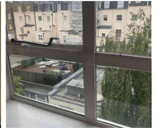
Figure 08: Existing Kitchen rear casement window.
