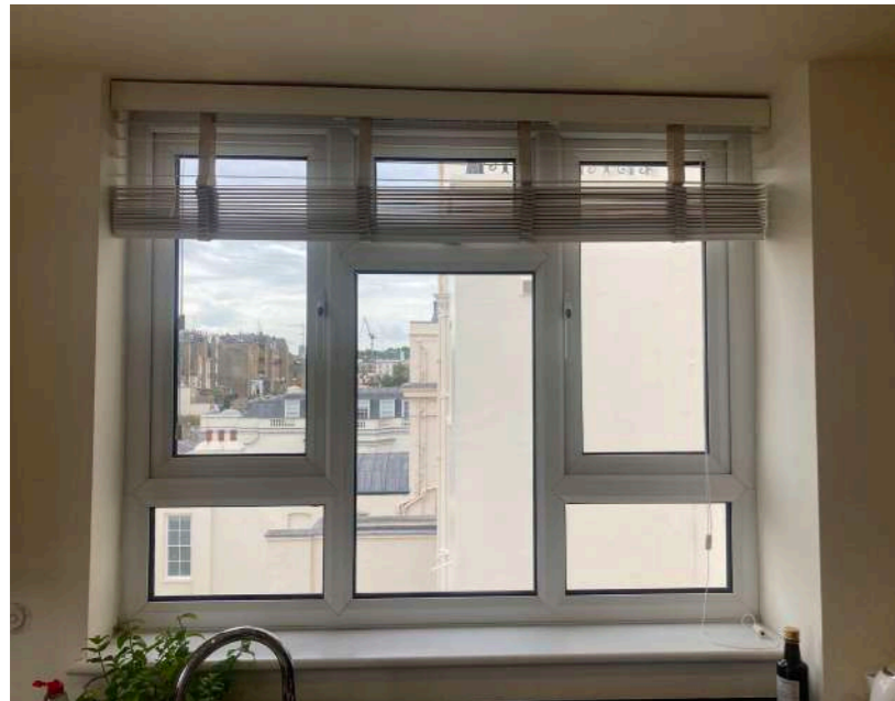
Figure 03: Existing Kitchen side elevation PVC double glazed casement window.
