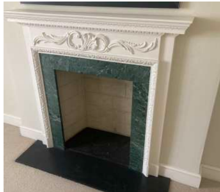
Figure 51: Existing Dining Room fire surround.
