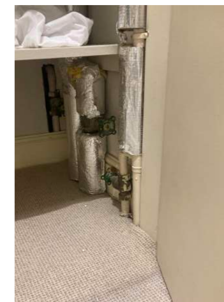
Figure 35: Existing drainage and plumbing within cupboard next to Bathroom 2.
