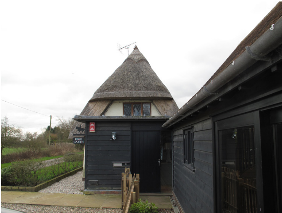
Existing main entrance
