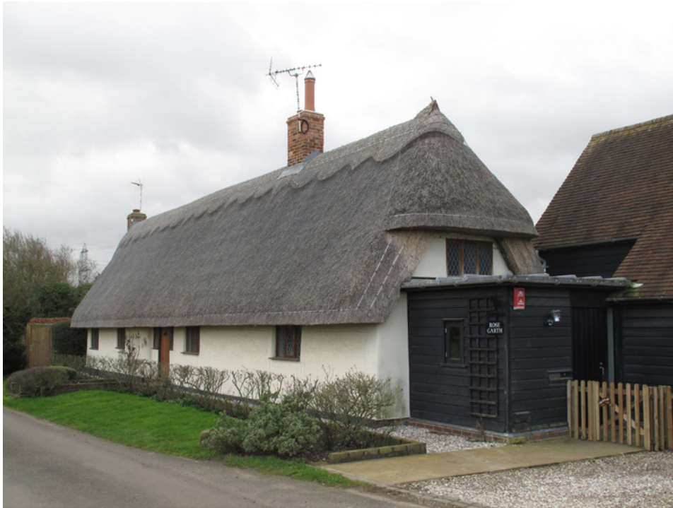
Existing main entrance street view
