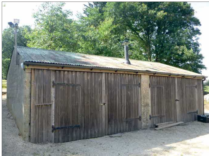
Photograph 3: Showing B2 scheduled to be demolished.
