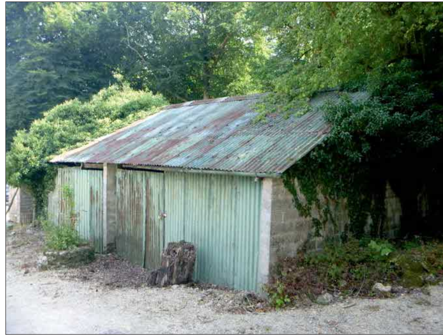
Photograph 2: Showing B1 scheduled to be demolished.
