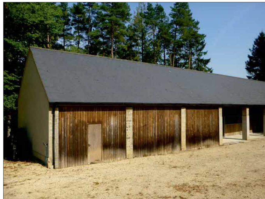
Photograph 4: Showing B5 scheduled to be retained.
