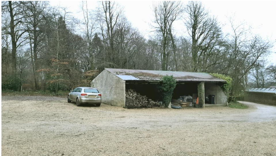
Site photo of Outbuilding B
